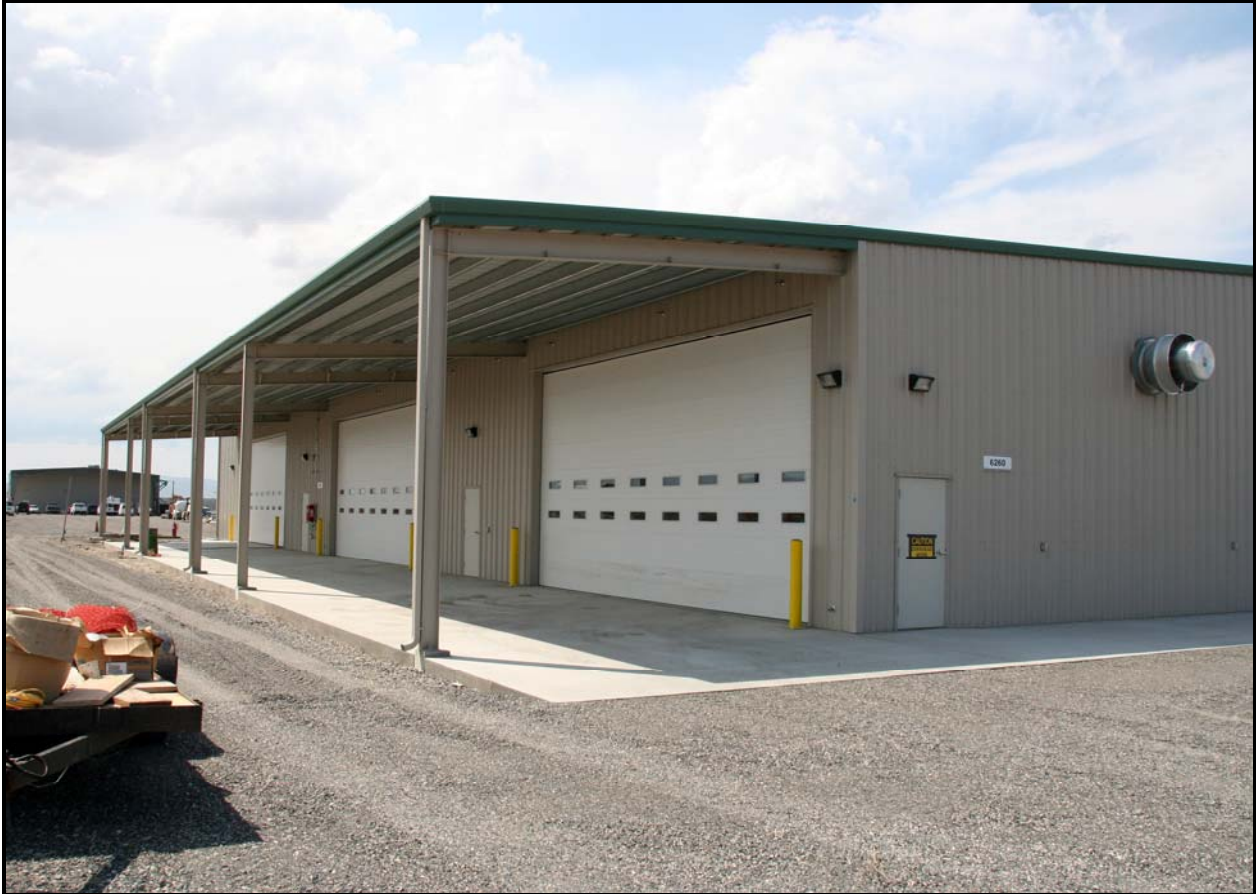
ERDF's new container maintenance facility includes three stalls, a repair line, a maintenance shop, and a weld area. (Photo 3)
