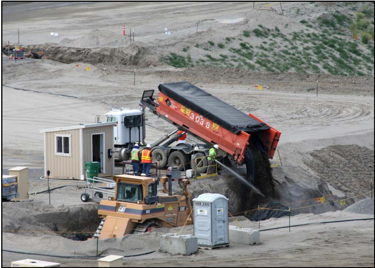
The waste disposal team used a new dump ramp constructed in super cell 9 at the Environmental Restoration Disposal Facility. (Photo 1)
