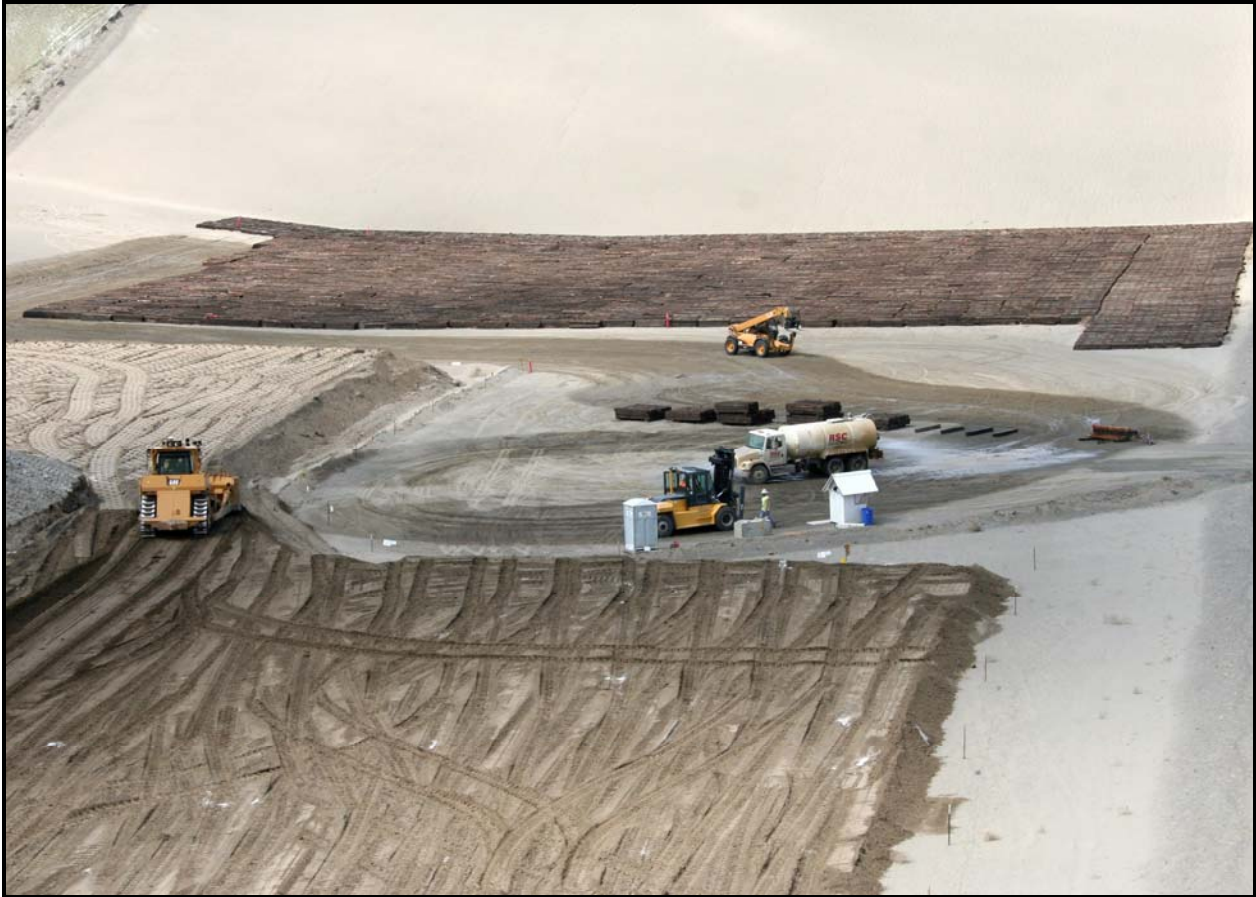
The waste disposal team spreads contaminated soil on the south side of super cell 9 while disposing railroad ties on the north side. (Photo 2)
