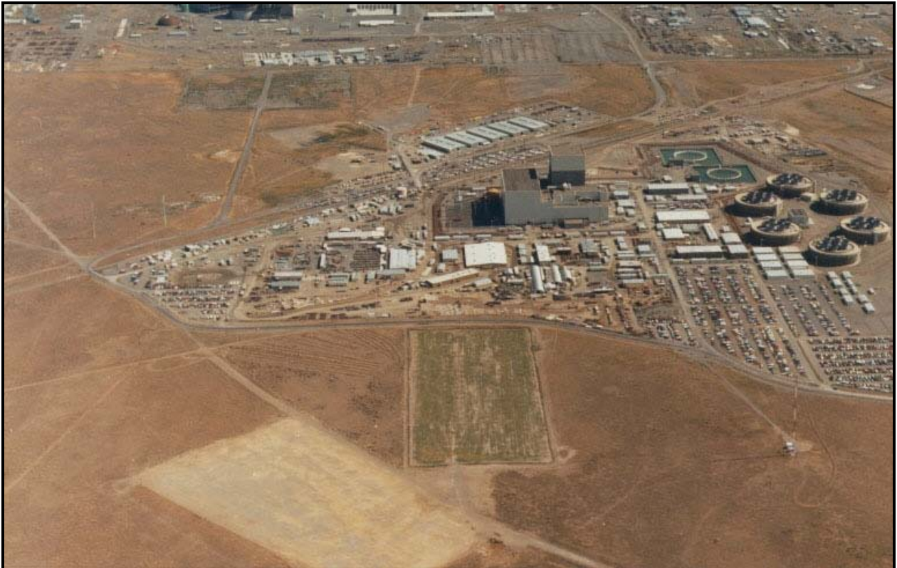
The 618-11 Burial Ground (green rectangle) is shown in this July 1998 photo. The site is adjacent to the Columbia Generating Station, a commercial nuclear plant. (Photo 7)
