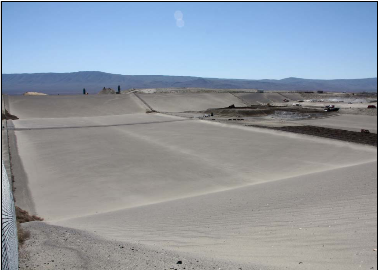
A view from the northeast corner of the Environmental Restoration Disposal Facility shows super cell 10 in the foreground and super cell 9, right. Waste is disposed in the south side of super cell 9, and railroad ties are being laid out on the north side. (Photo 1)
