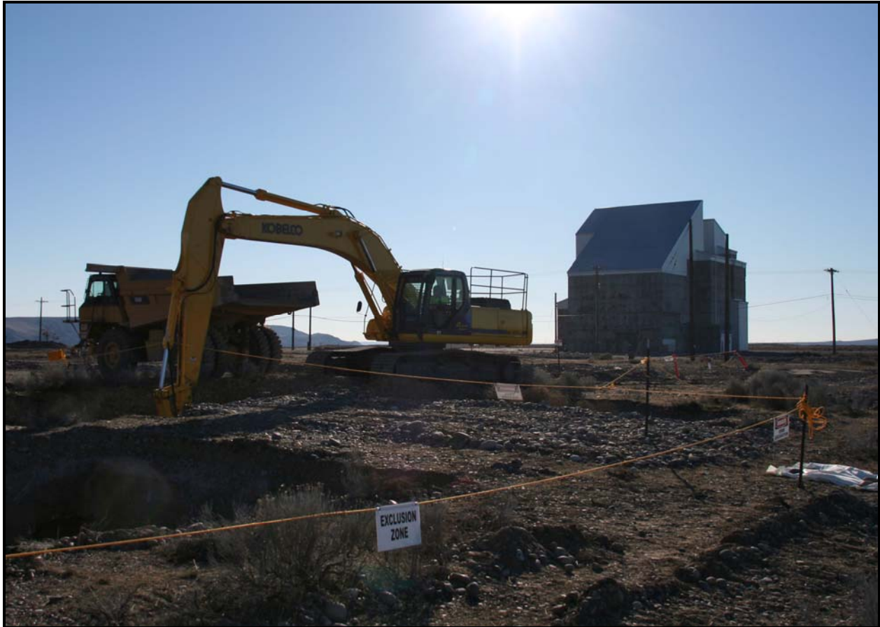
Washington Closure Hanford subcontractor Ojeda Business Ventures began loadout of stockpiled waste at 100-F-49, which contained a maintenance garage lube pit foundation. (Photo 9)
