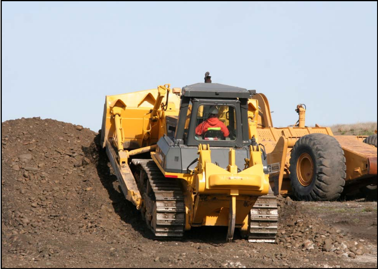
Work continues on the construction of roads at the 618-10 Burial Ground.
