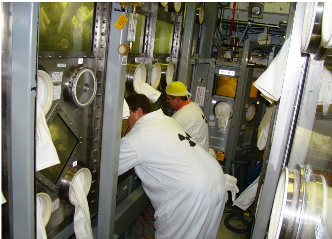
Workers perform decontamination on a glove box in the 234-5Z building.
