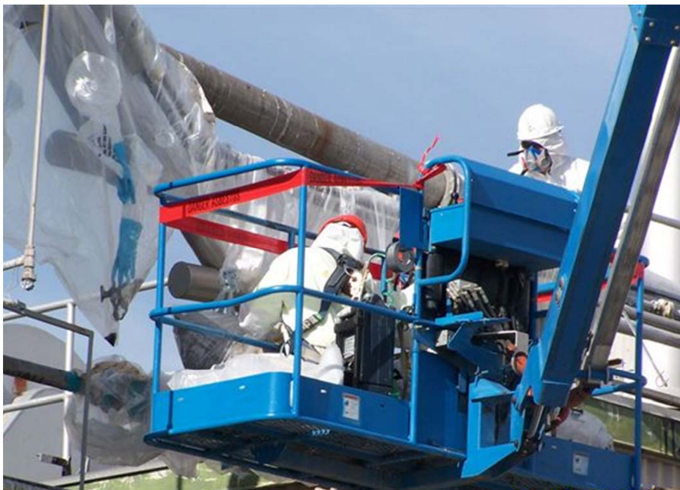
Workers are continuing to perform asbestos abatement on the 224-UA building.
