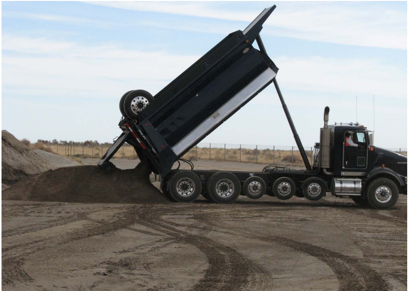
Workers participated in training exercises using clean dirt provided by personnel at ERDF.
