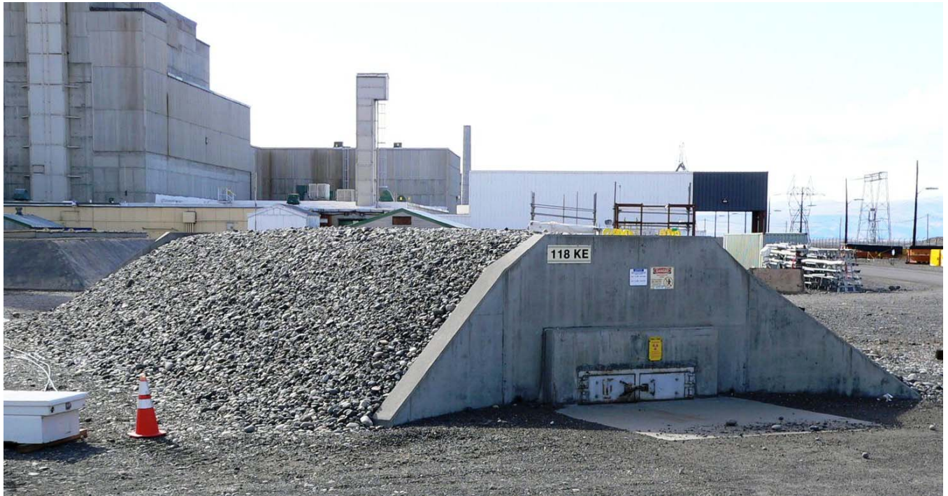
The 118KE Rod Storage Cave before D&D began. Several tons of gravel were removed earlier this year.
