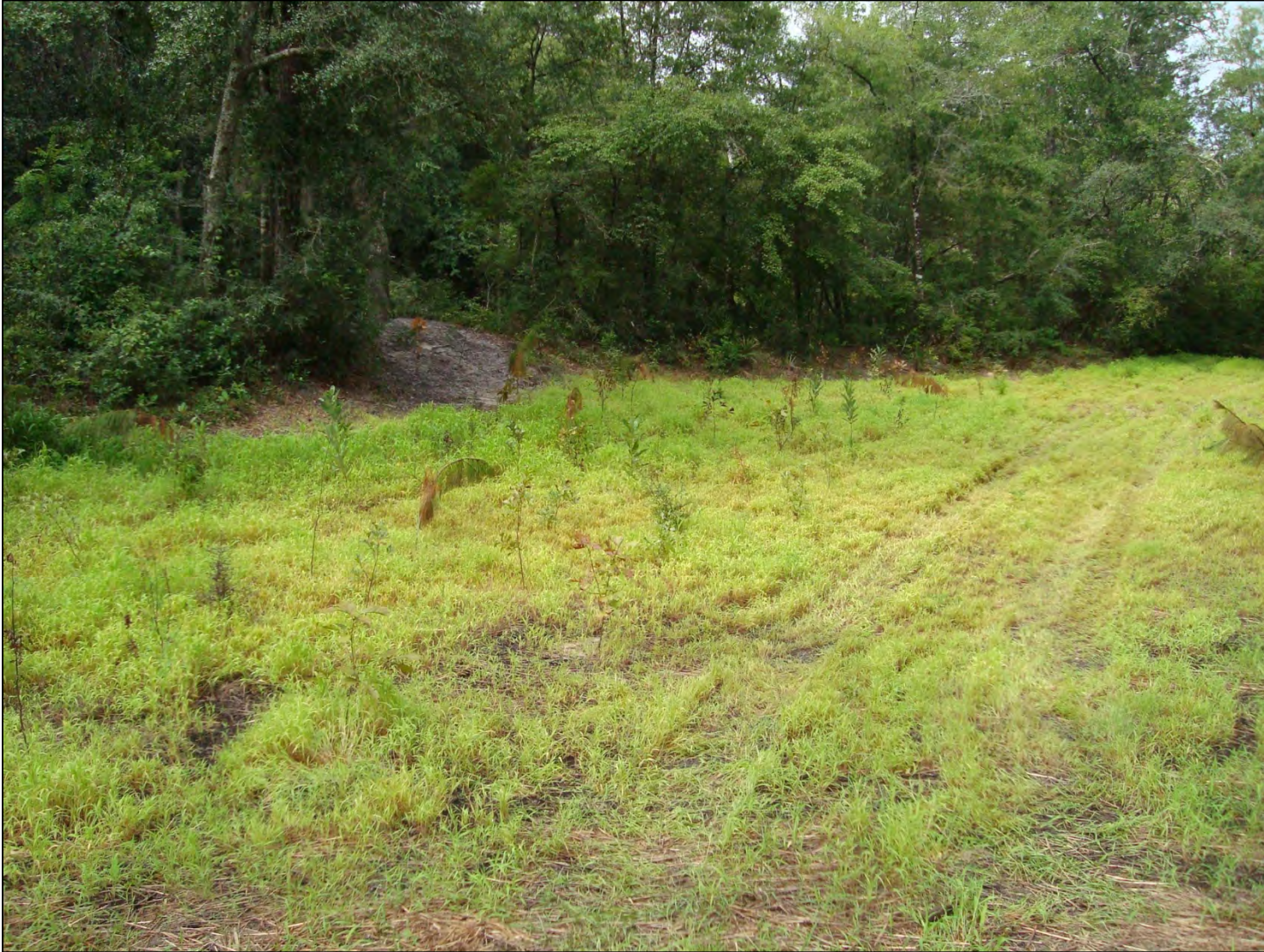
Figure 29. Unpaved road leading to Dripping Rock was stabilized by grading, filling, and seeding. Photo credit: The Nature Conservancy.
