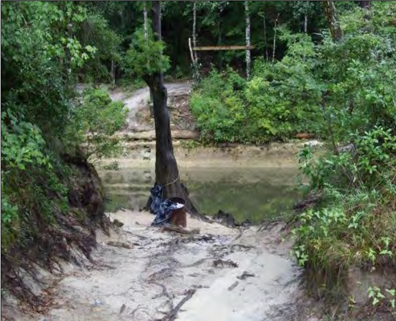
Figure 22. Denuded and breached riverbank at Dripping Rock. Photo credit: The Nature Conservancy.
