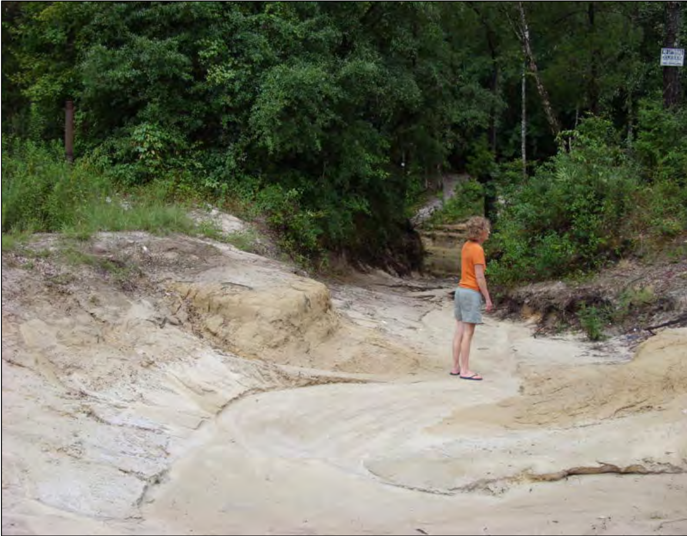
Figure 24. Unpaved road terminating at the denuded and breached riverbank at Dripping Rock. Photo credit: Eilene Beard.
