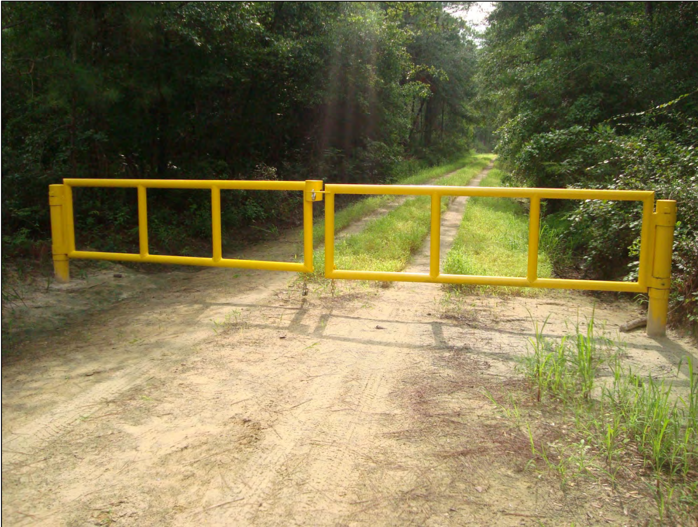
Figure 30. Heavy duty gate installed at entrance to unpaved road from Covington County Road 24 (Open Pond Road) to minimize continued human-induced degradation of the Dripping Rock area. Photo credit: The Nature Conservancy.
