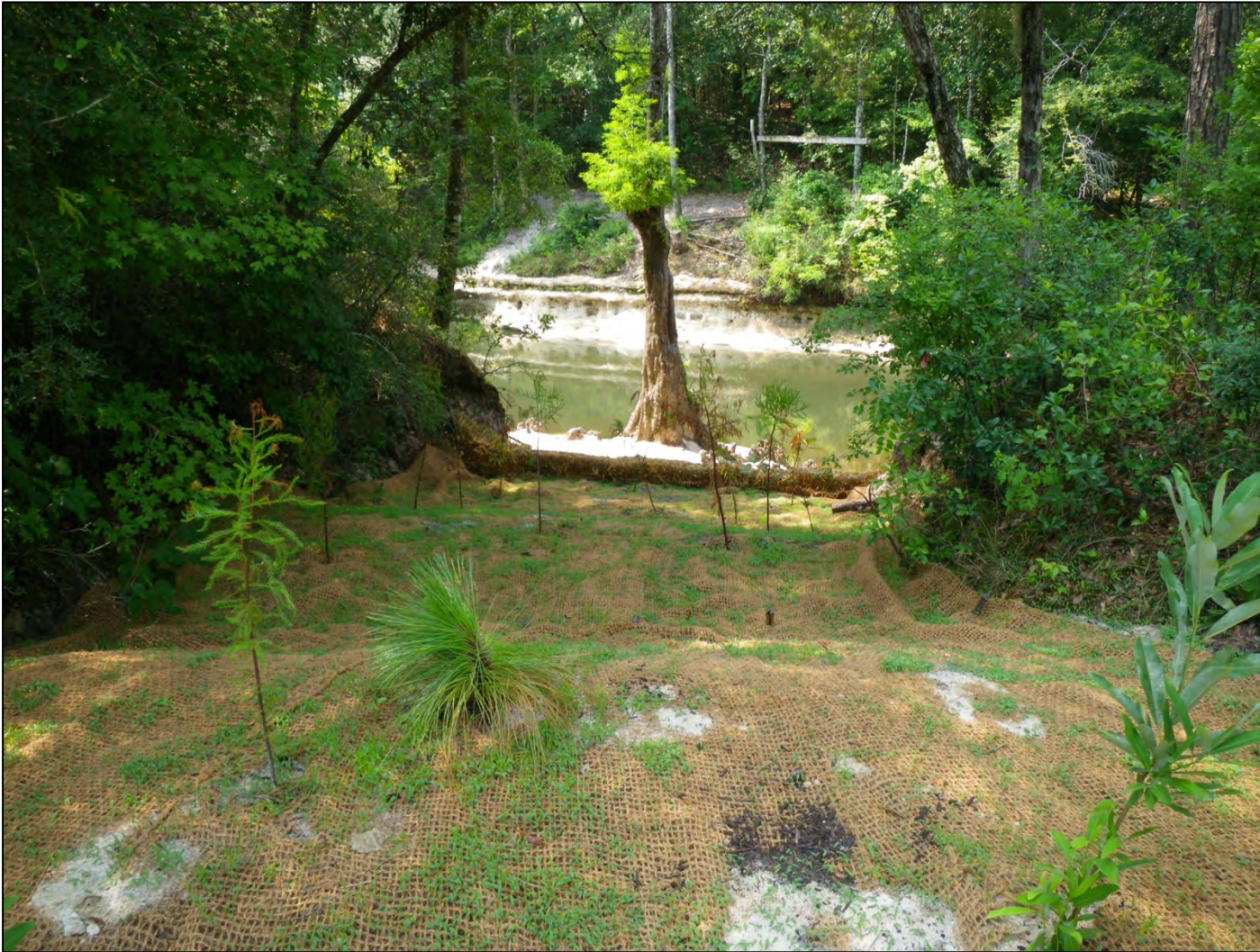
Figure 28. Restored river corridor showing a contoured terrace within the floodplain stabilized with native grasses, shrubs, and trees. Picture taken four days following restoration. Photo credit: U.S. Fish and Wildlife Service.
