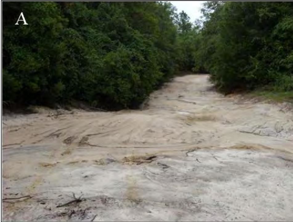
Figure 32. Comparison of condition of the unpaved road terminus at the breached riverbank, facing north towards the road, before (A) and after (B) restoration at Dripping Rock. Photo credit: The Nature Conservancy.
