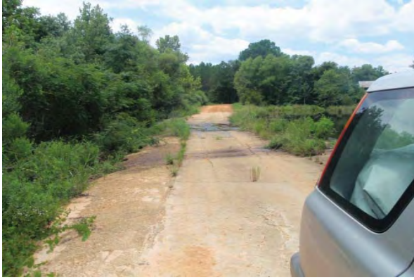
Crossing Structure: Lt Approach
