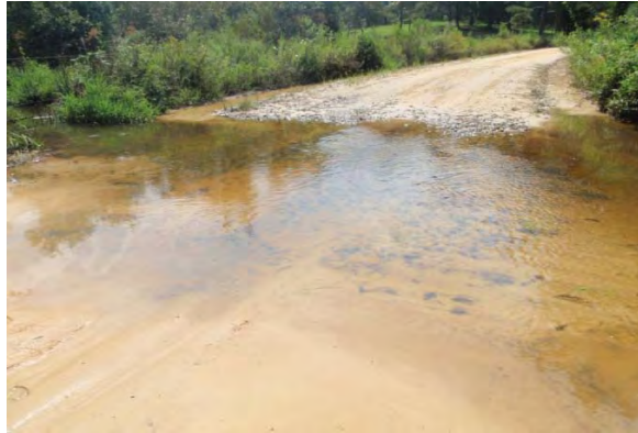
Crossing Structure: Rt Approach
