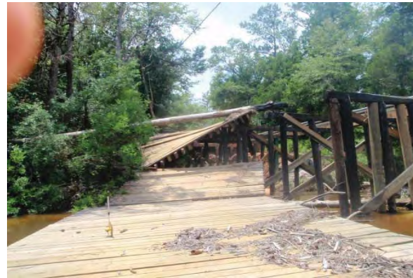
Crossing Structure- Rt Approach
