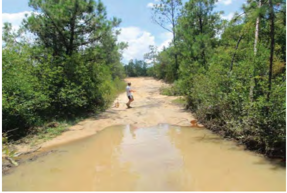
Crossing Structure: Lt Approach
