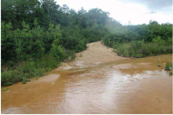
Crossing Structure: Rt Approach
