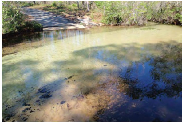
Crossing Structure: Rt Approach
