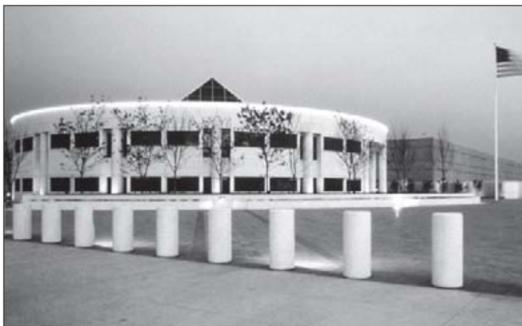
Western Currency Facility, Fort Worth, Texas.
