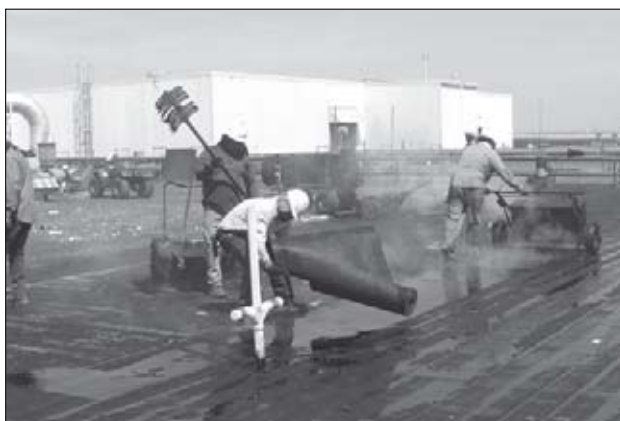
Workers prepare an area for installation of cool roofing material.
