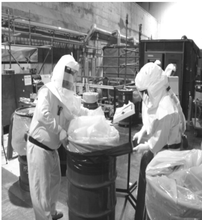
Nuclear chemical operators hired using Recovery Act funds prepare drums to be filled for repackaging at the T Plant Canyon.
