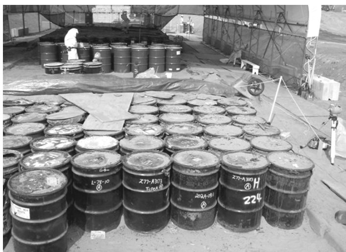
Retrievably stored waste removed from trenches awaiting shipment to a treatment/storage/disposal facility.
