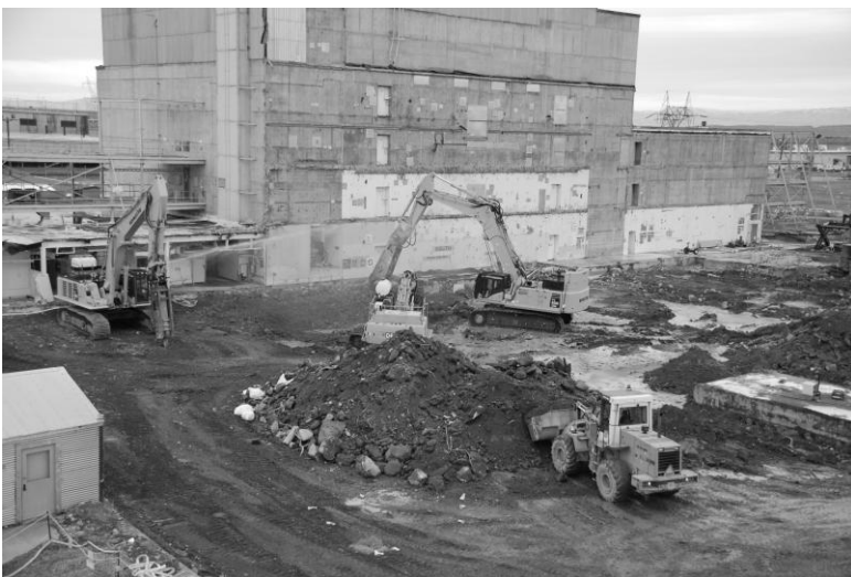
K East Basin substructure demolition
