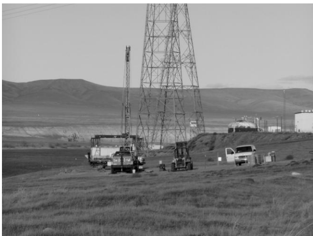
Groundwater well drilling in the River Corridor
