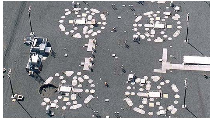
Aerial view of a Hanford Site tank farm
