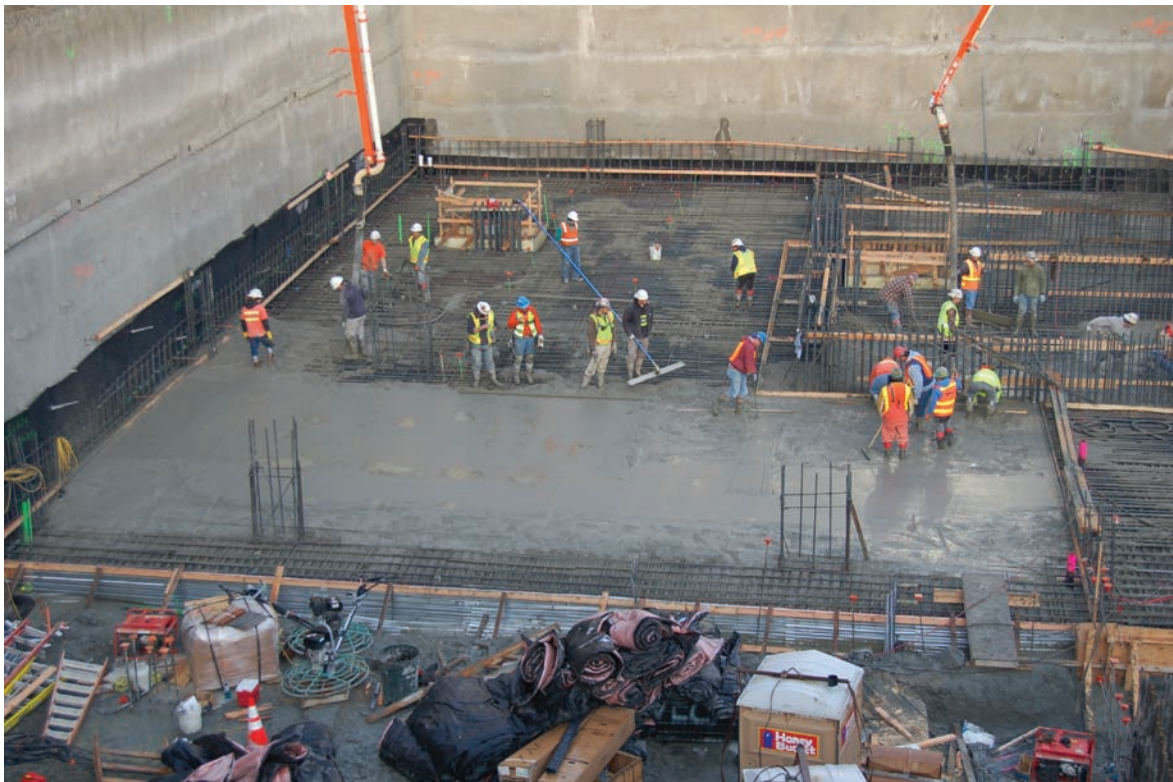
Figure 11-2 – A 10-ft thick mat foundation, pour in progress.
