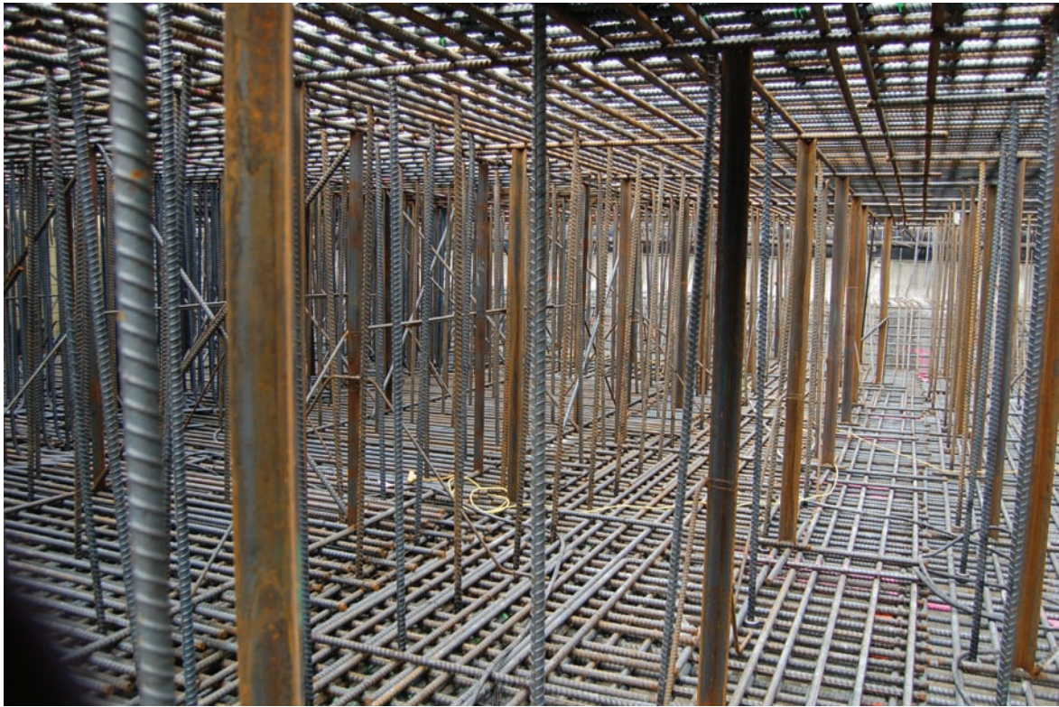
Figure 11-1 – Vertical reinforcement and steel angle standees.
