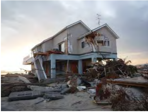
Photo 4.15 Remaining Mixed Building with Reinforced Concrete Piloti on First Floor
