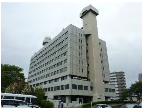
Photo 3.70 Overview of SI Building A
