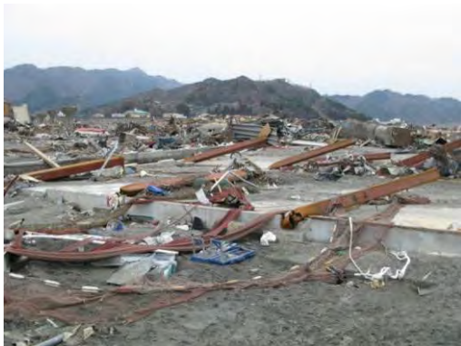
Photo 4.8 First-floor Columns Falling in the Same Direction
