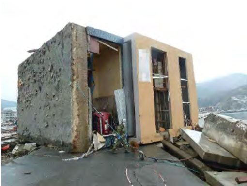
Photo 4.2 Overturning of 3-story Reinforced Concrete Building
