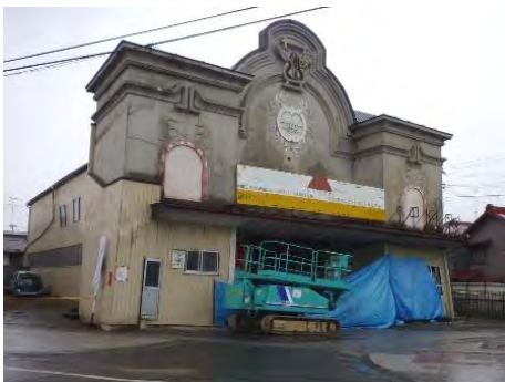
Photo 3.3 Large-scale Wood Building renovated to a Factory
