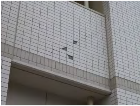
Photo 3.73 Drop of Ceramic Tiles
