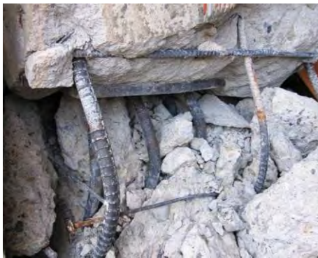
Photo 3.31 Close-up View of the Bottom of SRC Column
