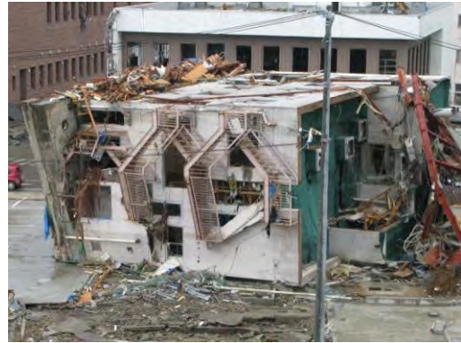
Photo 4.9 Overturning of 3-story Steel Building
