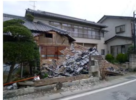
Photo 3.17 Breakage of Entrance Part
