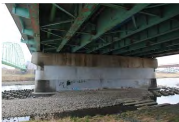
Photo 7 Retrofitted pier of Sendai Bridge which did not suffer damage during 2011 Great East Japan earthquake
