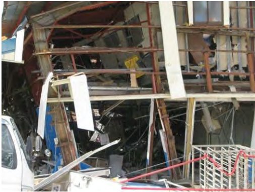
Photo 4.11 Tilted Gabled Roof Frame
