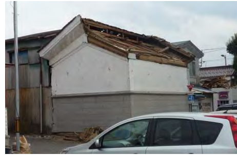
Photo 3.15 Fallen Roof Tile of Dozo
