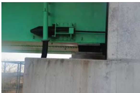
Photo 9 An end of deck supported by elastomeric bearings and unseating prevention devices
