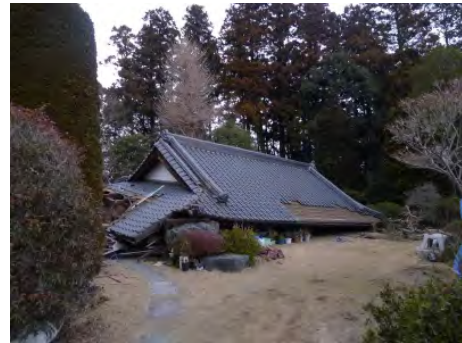
Photo 3.16 Collapsed Wood House
