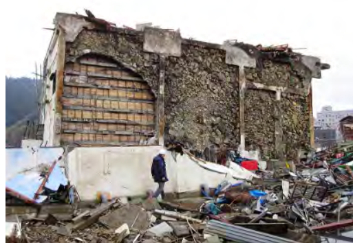
Photo 4.3 2-story Reinforced Concrete Building that Climbed over the Fence and Overturned
