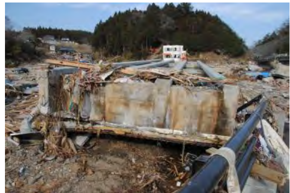
Photo 20 An overturned superstructure
