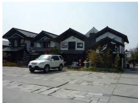
Photo 3.4 Warehouse with Mud Walls damaged Heavily or Slightly
