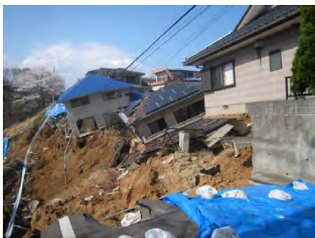
Photo 3.69 Land Sliding on Slope on the Southwest of the Hill and Sliding House
