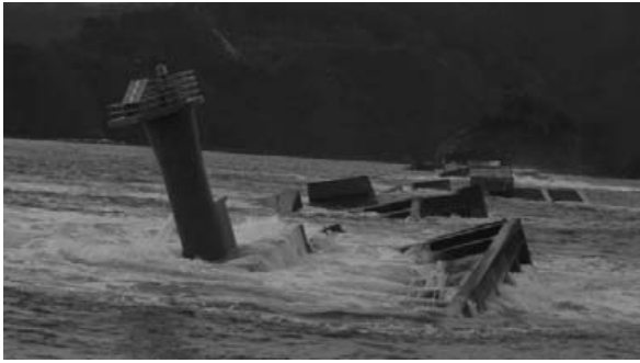
Fig. 9 Damaged offshore breakwater in Kamaishi Port
