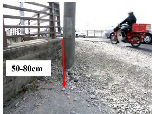
(c) Subsidence of Backfill soil of Abutment
