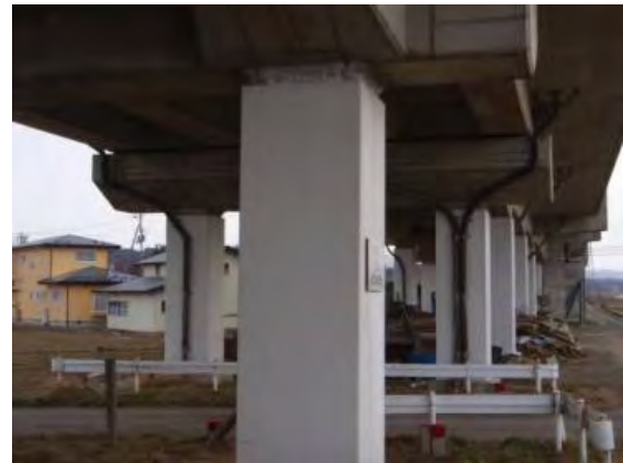
Photo 15 No. 3 Odaki viaducts which were retrofitted after 2003 Sanriku-Minami earthquake performed well during 2011 Great East Japan earthquake
