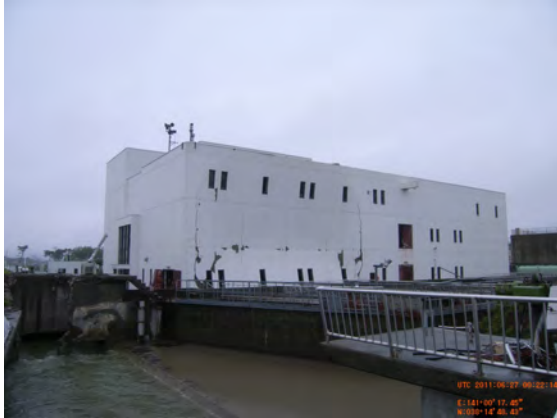
Figure 5 Minami Gamou Wastewater Treatment Plant Building.
