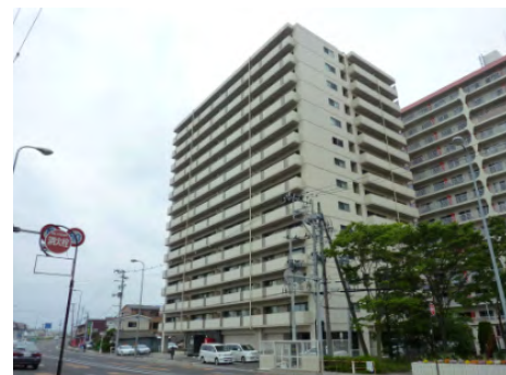
Photo 3.72 Overview of SI building B
