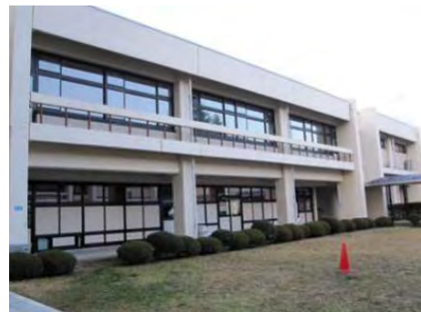
Photo 3.24 Appearance of Damaged Building
