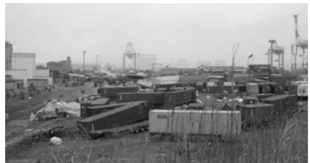
Fig. 13 Scattered shipping containers in Sendai-Shiogama Port
