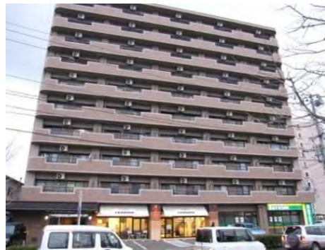
Photo 3.40 Appearance of Damaged Building
