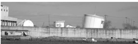
Fig. 6 Damaged oil tanks in Kuji Port
