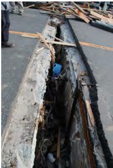
Photo 19 Effective restrainers to tie together adjacent decks
