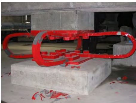
Photo 3.76 U-shape Steel Damper
