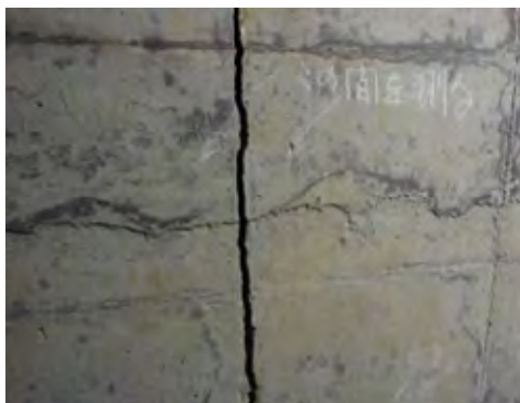
(a) Contraction joint 2J3
