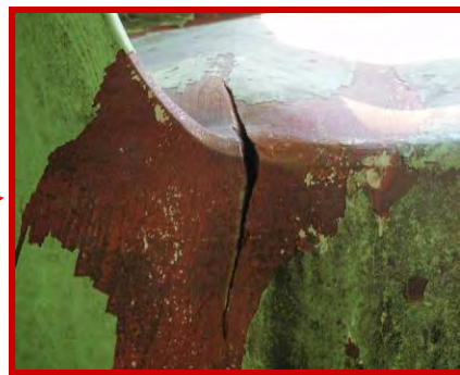
(e) Slight Buckling and Crack Observed in Lower Chord Member
