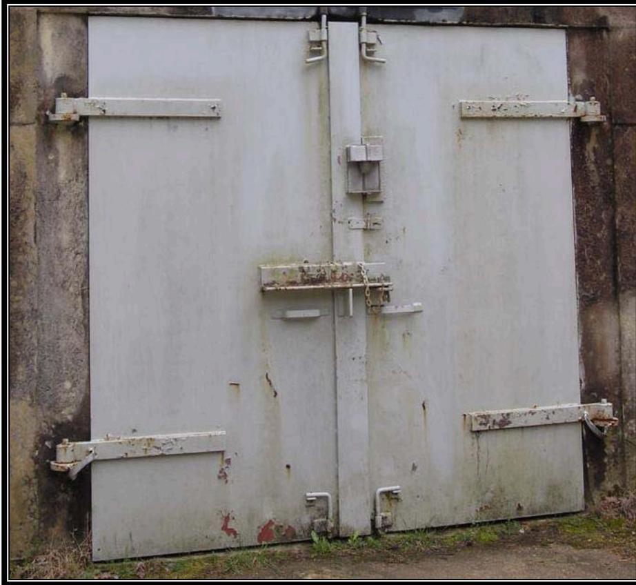
Plate 6.28 Typical igloo door, note ground straps on both lower hinges (Courtesy U.S. Army, 2007)
