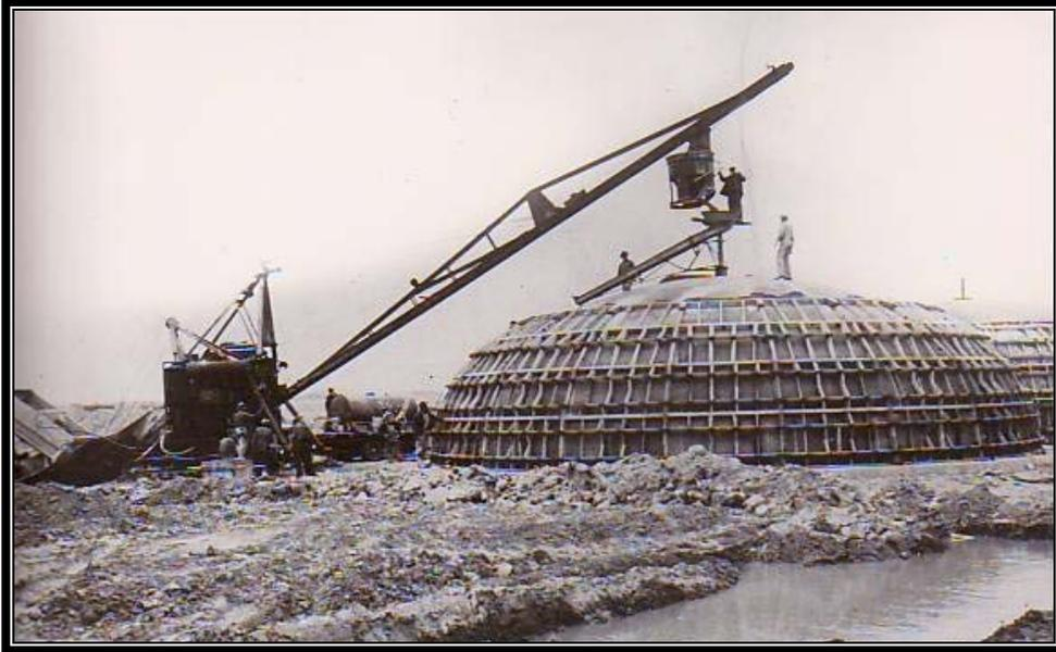
Plate 6.3 Corbetta Beehive under construction (Courtesy U.S. Army)
