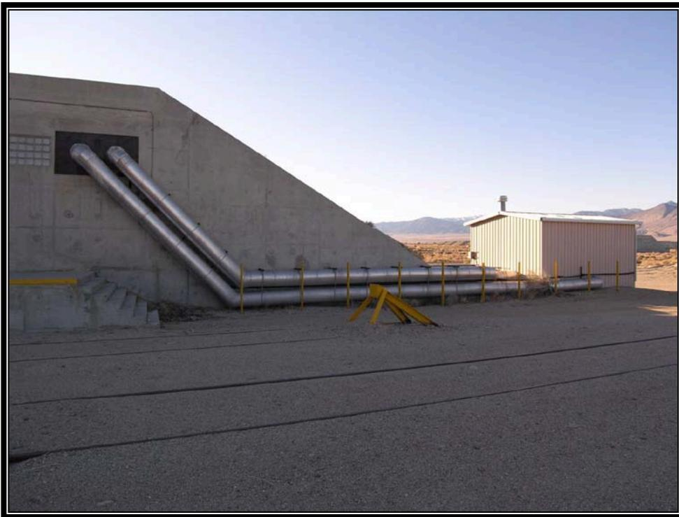
Plate 7.15 Typical earth-covered magazine modified with heating plant to create a constant temperature magazine (Courtesy U.S. Army, 2007)
