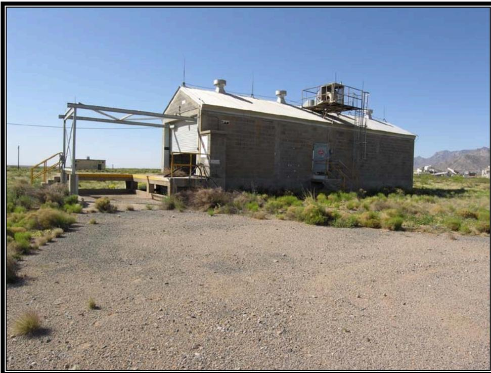
Plate 6.12 Liquid propellant storage building, note lightning rods (Courtesy U.S. Army, 2007)
