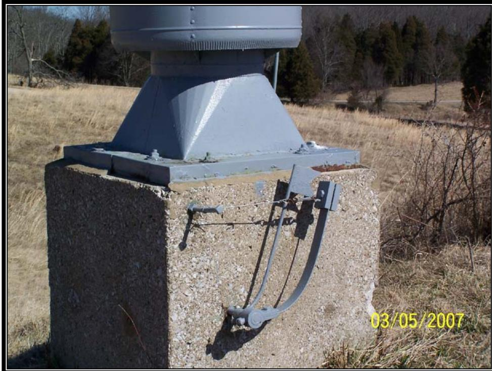
Plate 7.18 Detail of typical igloo ventilator. Note counterweight and flag that would pop-up if ventilator closed (Courtesy U.S. Army, 2007)
