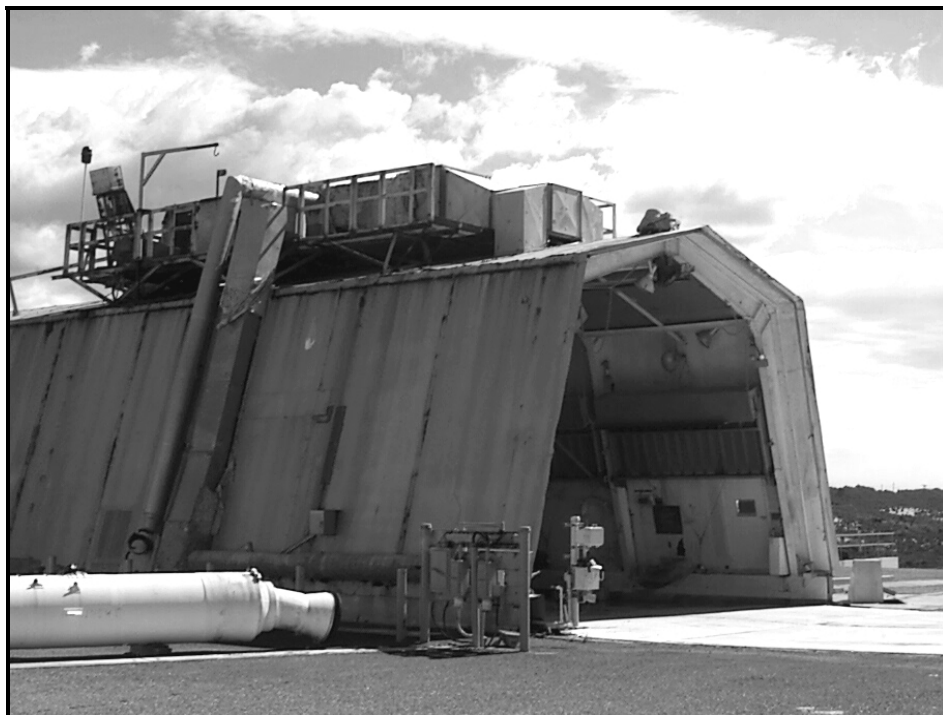
Figure 48: View of West End Shelter. Note air conditioning units on top of Shelter and the Clean Air Monitoring Station (small metal box below center on Shelter wall)
