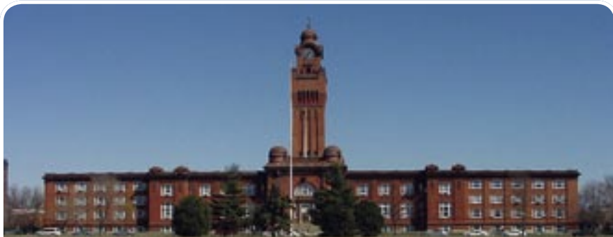
Naval Station Great Lakes, Building 1 Administrative Building – Headquarters: Courtesy of Naval Station Great Lakes
