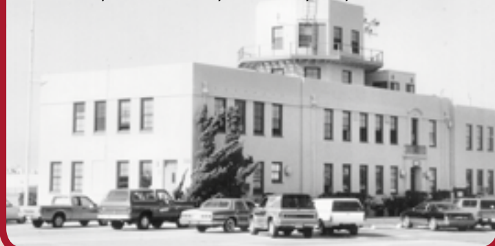
Control Tower, Naval Air Station, North Island, Calif., 1930s
