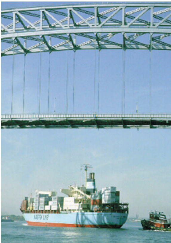
A container vessel navigates the Kill Van Kull channel as it passes under the Bayonne Bridge, N.J. The Corps has deepened this channel to accommodate modern shipping vessels.
