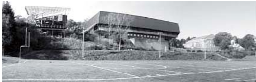
Visitor's Center, Roland Field House, Billard Gym
