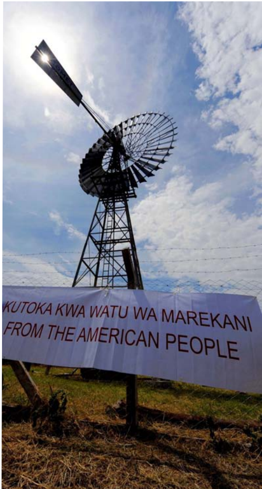
MAGU, Tanzania — A windmill connected to seven wells was the focal point of a water dedication ceremony January 21, 2009. The Magu water project provides clean drinking water to thousands of residents in the Magu region of Tanzania and is an example of how Combined Joint Task Force - Horn of Africa develops partnerships to promote regional cooperation and an environment for development. (U.S. Air Force Photo by Staff Sergeant Joseph L. Swafford Jr.)
