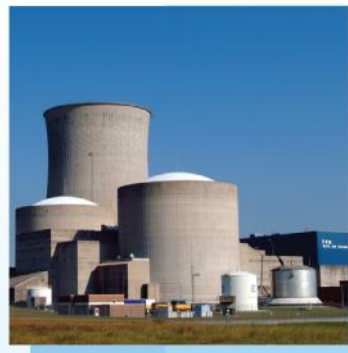
Power uprates and plant life extension
