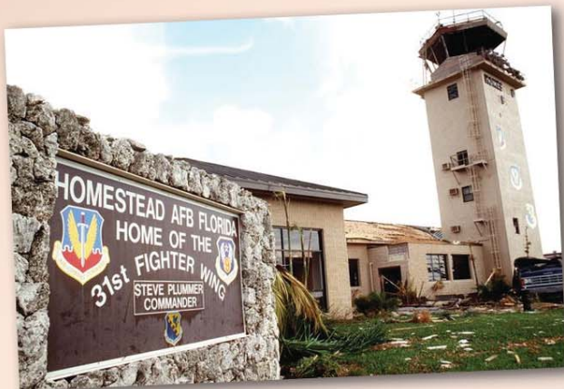
August 1992: Damaged control tower and welcome sign at Homestead AFB, Fla. Hurricane Andrew drove through the air base damaging every building on the base. Photo by Master Sgt. James Ferguson
