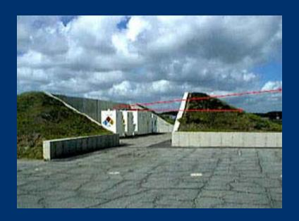
When evaluating whether a magazine is properly barricaded to a highway, determine whether a straight line, from the top of any side wall of the magazine to a point 12 feet above the center of a highway, will pass through the barricade.
