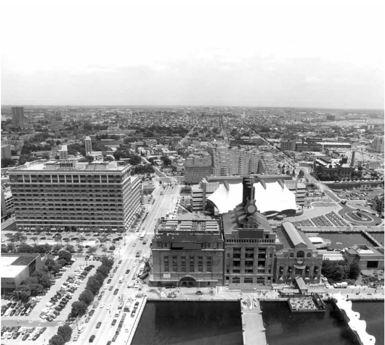
Office buildings, industries, residences, and transport systems, Baltimore, Maryland; east view from the inner harbor. Source: U.S. Department of Energy.
