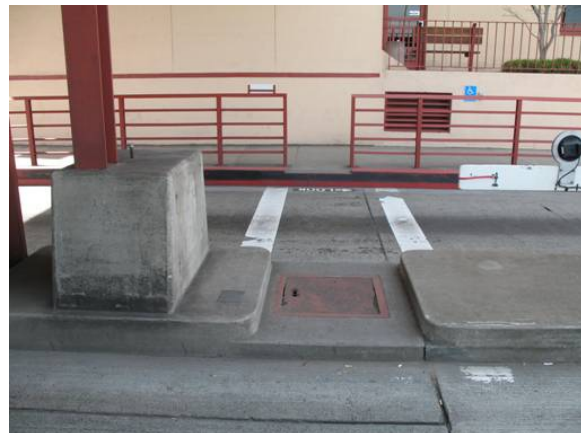
Figure 4-10. Painted Crosswalk for Workers with Fencing to Channelize Workers to Cross at the Crosswalk
