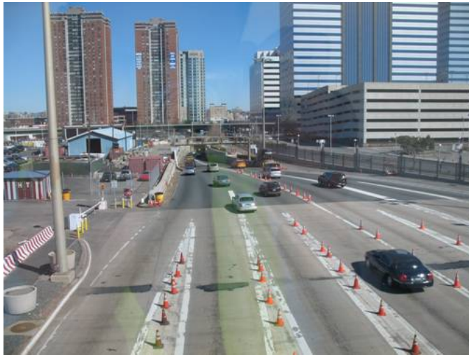
Figure 4-3. Pavement Markings and Cones Delay Merging Downstream at the NYS Thruway's Holland Tunnel Plaza
