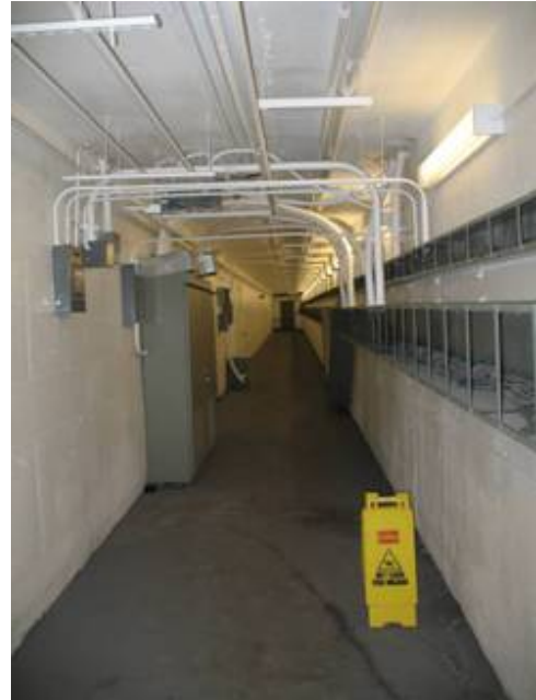
Figure 4-6. Tunnels Provide Access to Booths without Exposure to Traffic
