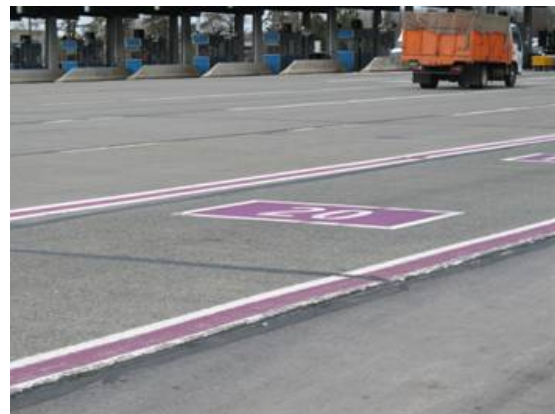
Figure 4-25. Pavement Markings Reinforce the Speed Limit in Dedicated ETC Lanes
