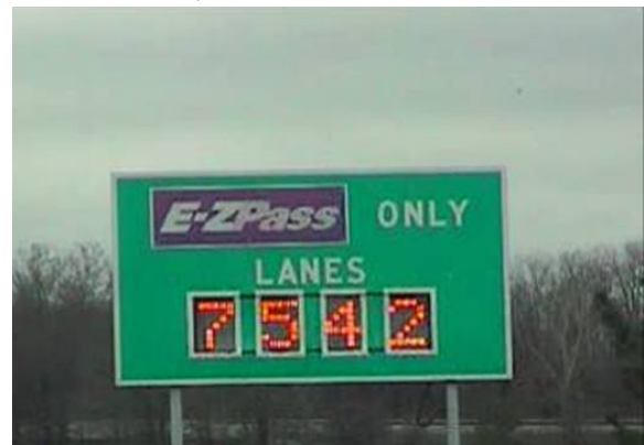
Figure 4-20. Dynamic Signs Display Current ETC Lane Numbers at a NYS Thruway Plaza
