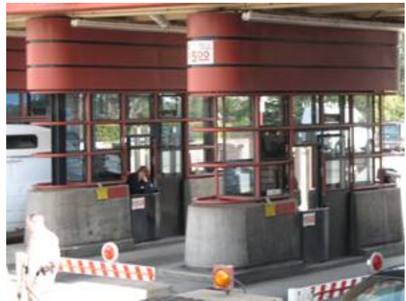
Figure 4-21. Gates in use to Indicate that a Lane is Closed
