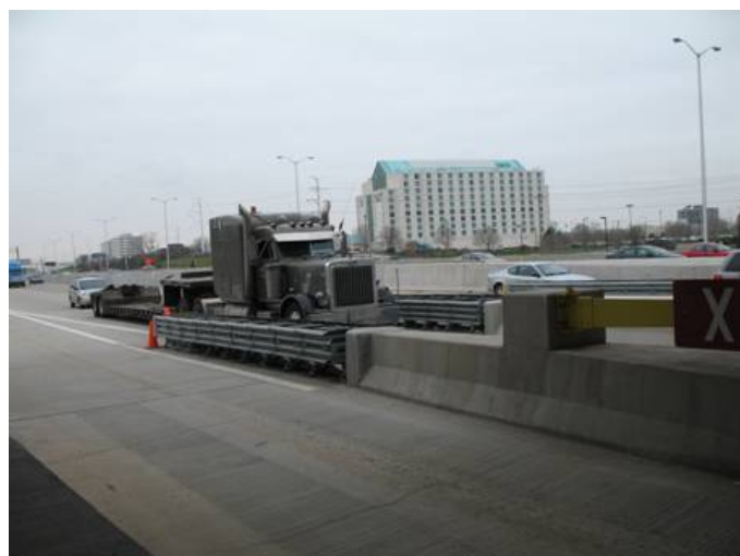
Figure 4-2. Concrete Barriers and Attenuators Physically Separate Traffic Upstream of an Illinois Tollway Plaza
