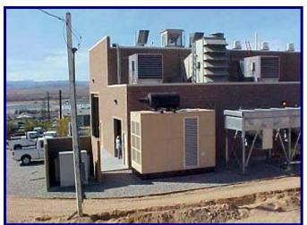
The Marine Corps saves \$5.8 million annually with this 7.2-MW, dual-fuel cogen system. ORNL's review of project plans resulted in improvements in the system's efficiency.
