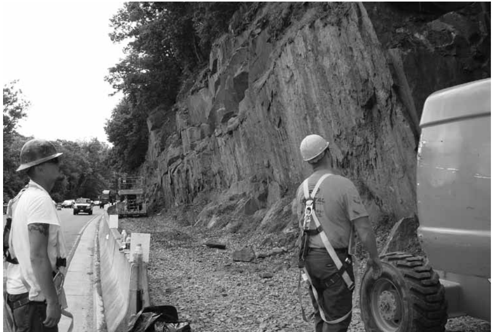
A rock cut slope on the George Washington Memorial Parkway in Arlington, VA.
