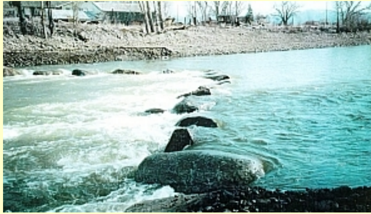
Vortex rock weirs,completed installation, Carson River, 1999
