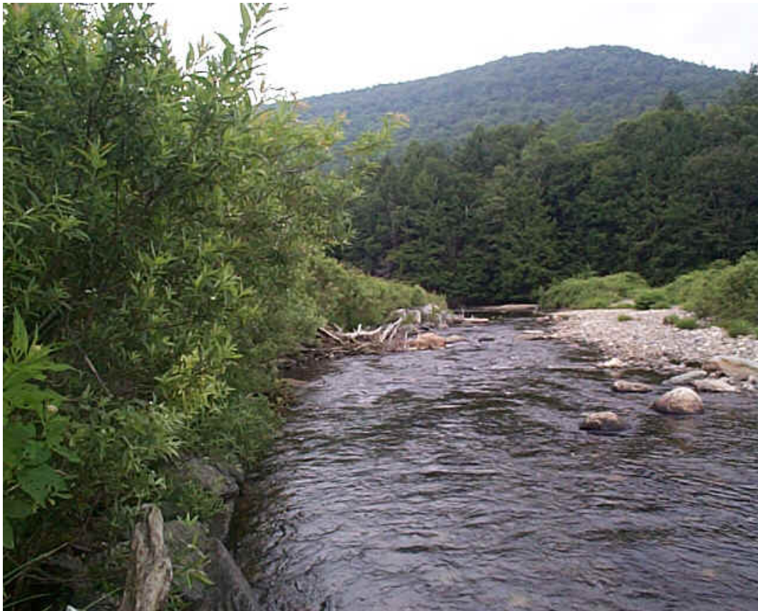
Down stream view - willows have overgrown rock revetment
