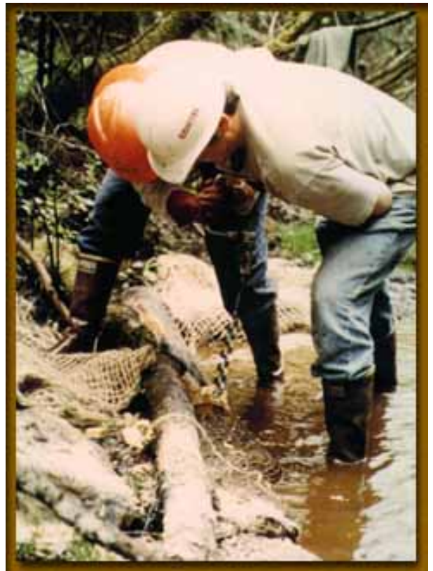
Americorps volunteers installed wood log structures, sand bags, jute matting, and planted willow stakes to improve the riparian corridor, reconfigure the stream banks and channel and improve the sinuosity of this reach of Duck Creek in order to improve salmon spawning habitat.
