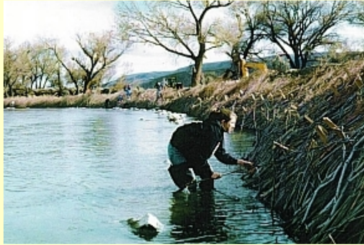
Placing dormant willow cuttings for soil bioengineered bank stabilization
