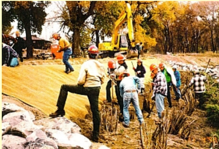
Coconut Fabric (Coir) Erosion Control Placement, with willow root ball planting and seeding, Carson River, 1998
