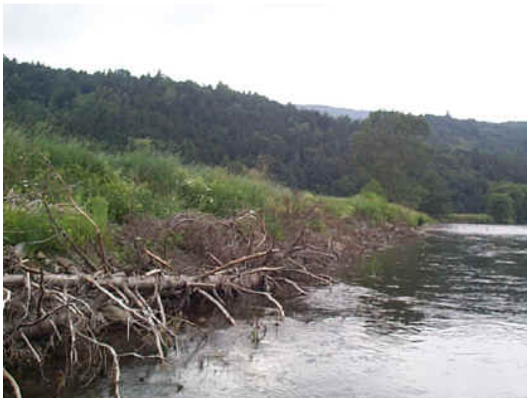
Tree revetments stabilizing toe of bank after 1 year
