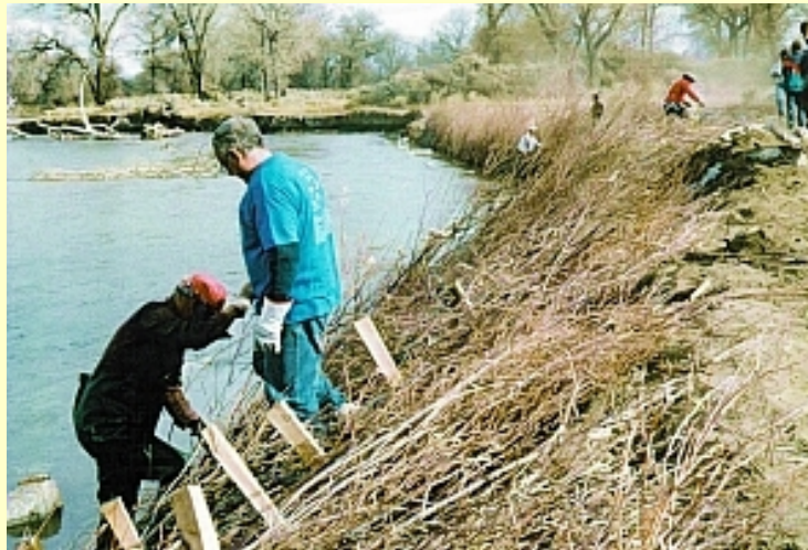
12 gauge smooth wire being installed to secure dormant willow cuttings
