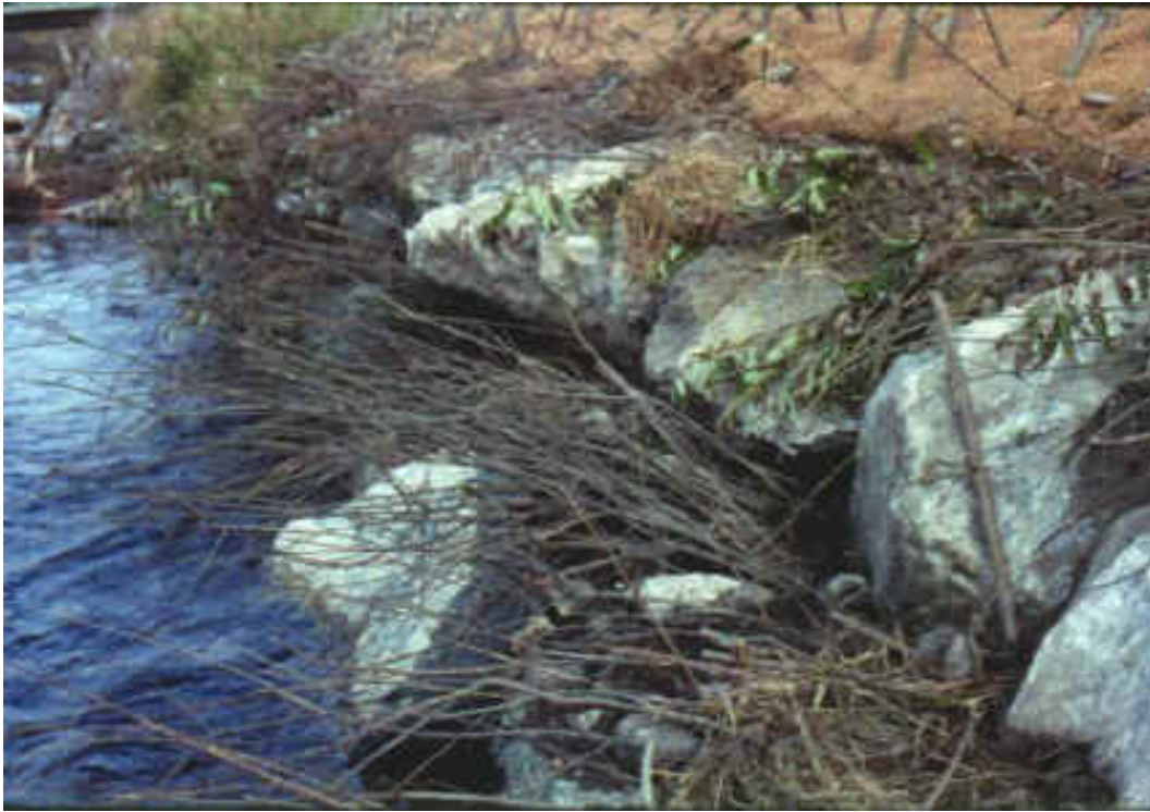
Close-up of rock revetment with brush layers
