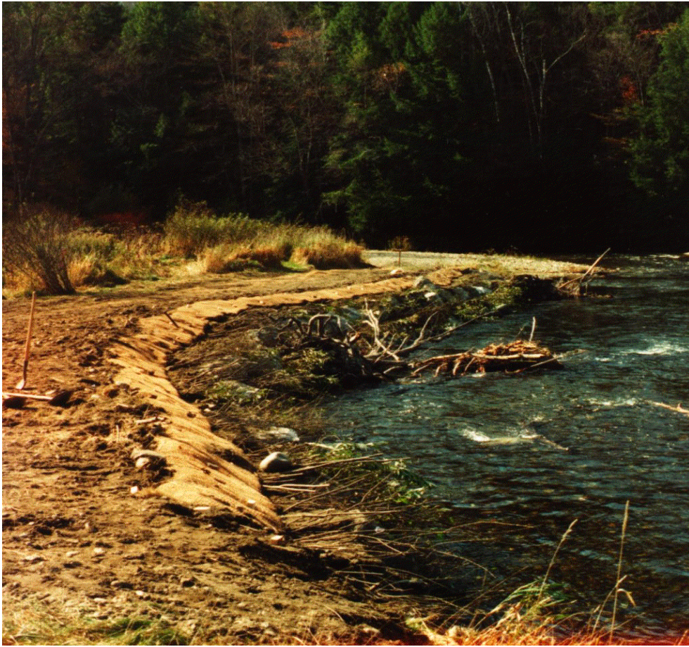
Down stream immediately after installation
