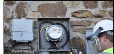
OG&E smart meter installation
