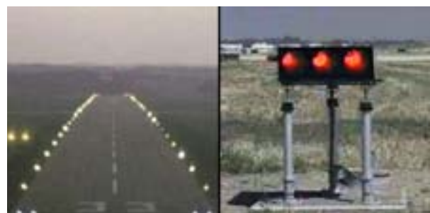
Figure 16: FAROS System PAPI Lights
