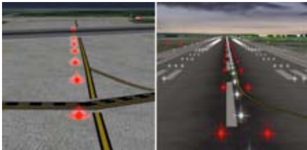
Figure 14: Runway Status Lights
