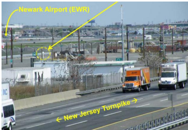
Figure 5: In Harm's Way -- FAA GBAS Installation at EWR
