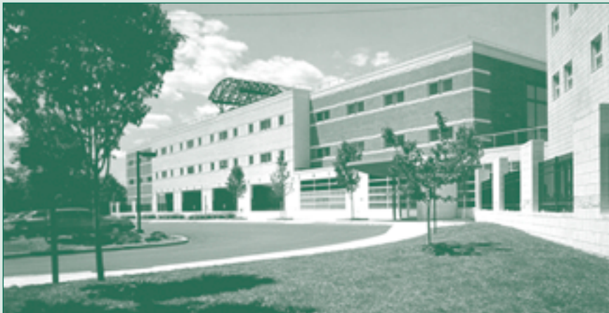
Dutchess County Jail Facility, Poughkeepsie, New York. Ricci Greene Associates, Design Architect • Gruzen Samton, PC, Architect of Record
