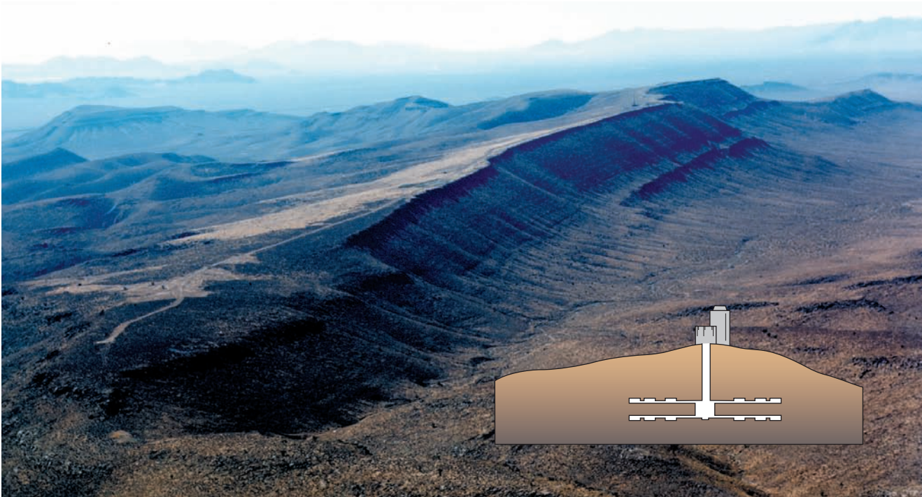
Figure 2. The Planned Nuclear Waste Repository at Yucca Mountain The planned geologic repository at Yucca Mountain, Nevada, is designed to hold 63,000 tonnes of commercial spent nuclear fuel. A decision on a second repository is needed by 2010 in order to keep pace with the accumulation of waste. The inset suggests the many tunnels belowground that will house the waste.
