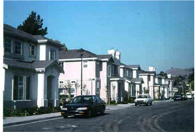
Undesirable: The use of a single palette of colors has assisted in creating monotony and an appearance that all the homes are the same throughout a development.
