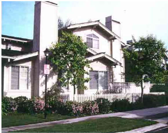
Desirable: Articulation of elements along corner lot sideyard should be comparable to front yard building articulation.
