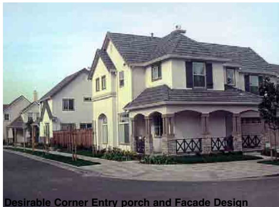
Desirable Corner Entry porch and Facade Design
