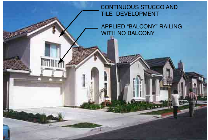
Undesirable: Recent developments have been nearly all of a single material, stucco, creating monotony. Also, detailing or “applied” materials are used inappropriately.
