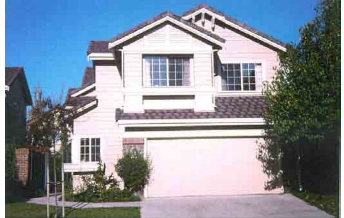
Recent small lot single family developments have placed large, standard sized homes on the small lots. The Planning Commission and City Council have each noted that the homes appear too large for the small lots.
