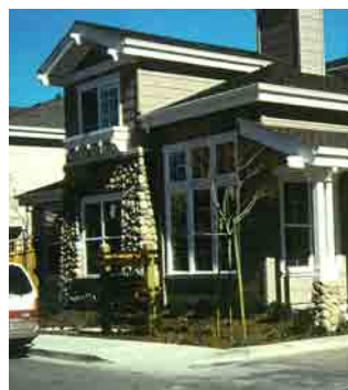
Desirable: Corner lots which orient entries and extend architectural detailing to all visible elevations.
