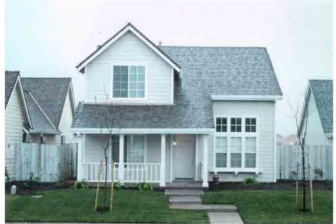
Desirable: Front Yard without garage or parking apron
