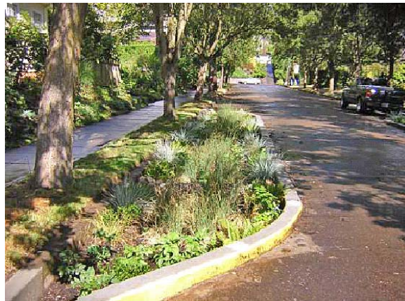
Exhibit 4.20: Stormwater curb extensions are functional and attractive additions to a streetscape. Street runoff flows into the landscaping and soaks into the ground.
