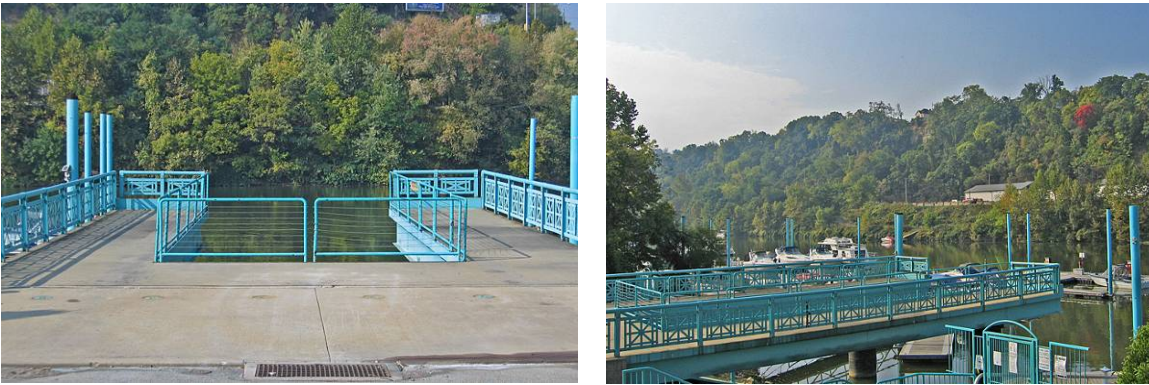
Exhibit 4.11: In McKeesport, Pennsylvania, this boat launch doubles as a public walkway when the lift below is not in use
