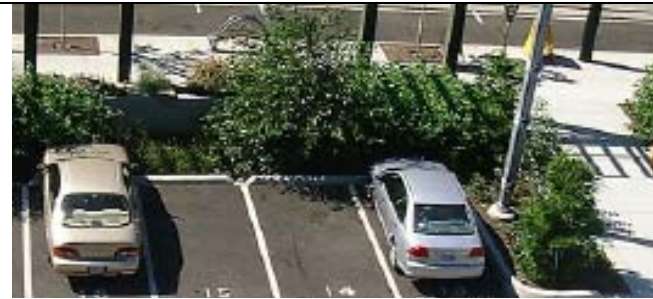
Exhibit 4.9: This parking lot retrofit (upper image) and parking lot basin (lower), demonstrate how adding infiltration basins requires little space and adds more greenery to the streetscape
