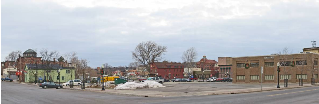
Exhibit 4.13: The top image is a view of Baraga Avenue and Front Street in downtown Marquette. The bottom is a design possibility that emulates a well-designed parking structure from Staunton, Virginia, which would break up the large greybelt and make the area a nicer place to walk.
