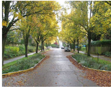
Figure 19 - Example of stormwater treatment along a planting strip Credit: Dover, Kohl & Partners
