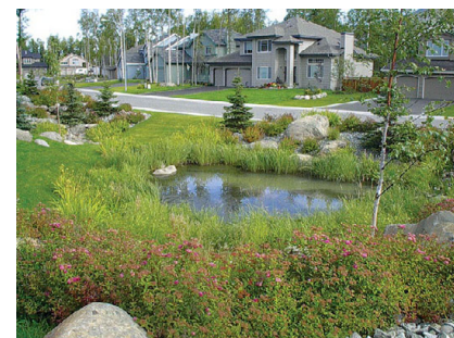
Figure 25 - Example of a rain garden Credit: www.swarthmorepa.org
