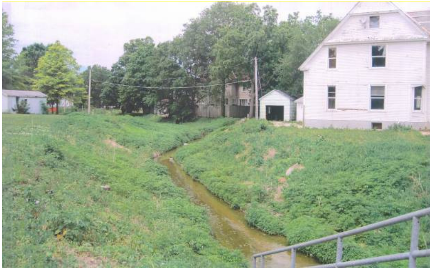
Figure 46 - Existing conditions. A photograph of Dry Run Creek in its existing form. Credit: FEMA
