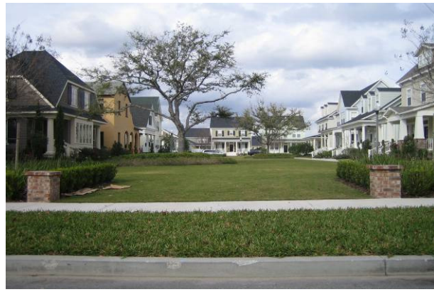
Figure 56 - Single family homes around a common green space Credit: Dover, Kohl & Partners
