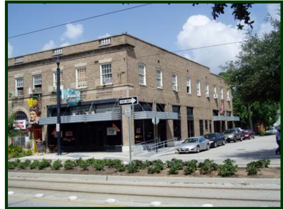
Figure C-12. Example of Missing Crosswalk
