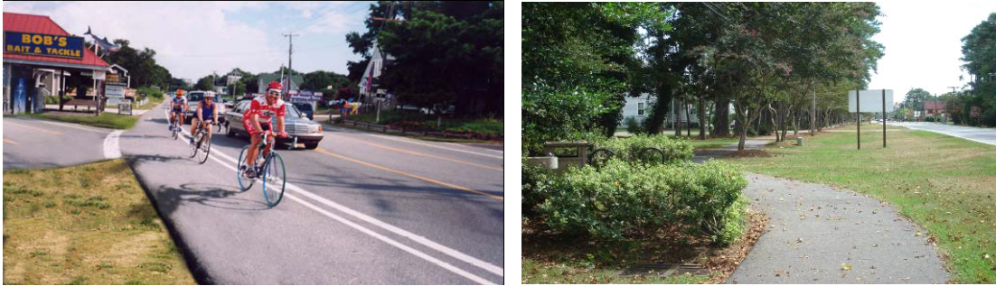
Figure 45. Wide paved shoulder/bike lane in Duck on NC Hwy 12 (left). Side path along U.S. Hwy 64/264 in Manteo (right). 60
