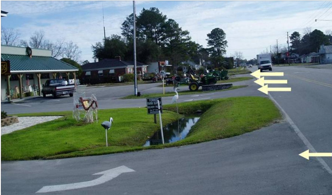
Figure 16. Four driveways along a segment of Hwy 55 in Bayboro. The business on the left has three points of access to the highway (two from the front and one from the side). Sharing access with the adjacent parcel (foreground) or limiting access to a side street (the top arrow indicates the position of a local street that connects to Hwy 55) would reduce two or three highway access points featured in this photo. 25
