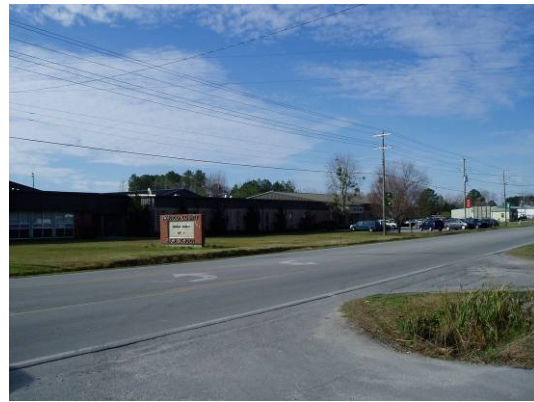
Figure 44. Pamlico County High School. Hwy 55 in the foreground. 58
