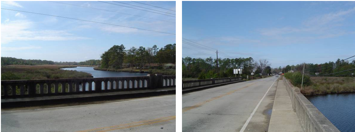
Figure 3. The communities of Bayboro and Stonewall share a gateway that consists of structural and natural elements in the form of the Bay River and the bridge traversing it. 6
