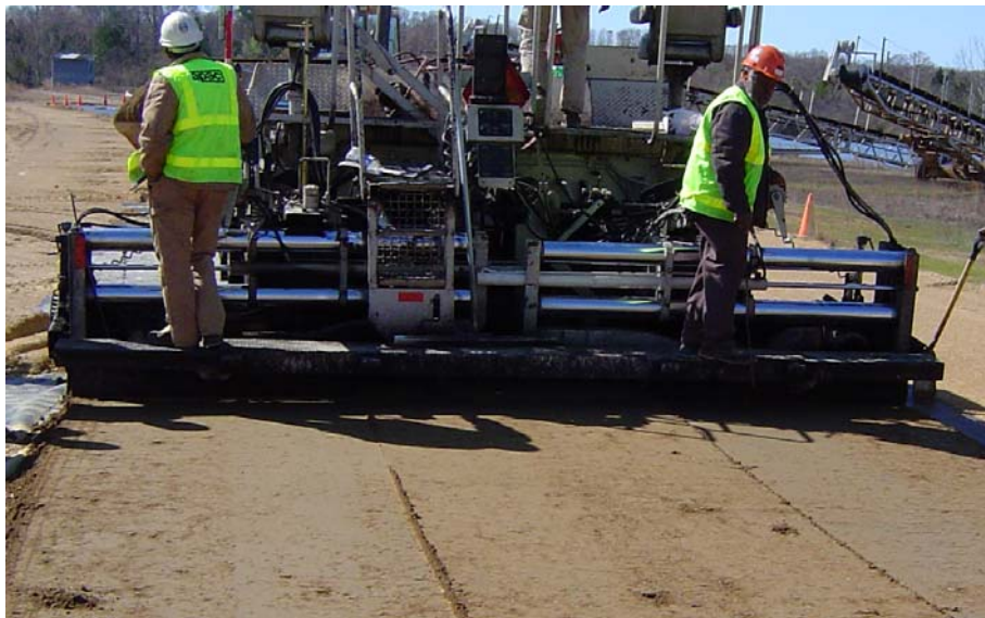
Figure 4-1. CTB placement with an asphalt paver.
