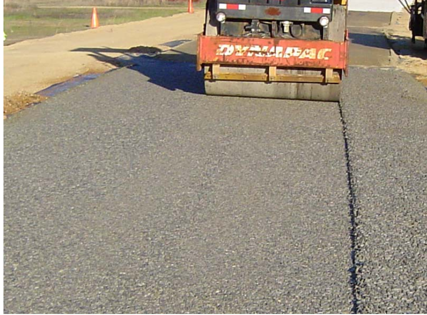
Figure 4-2. CTPB compaction with a static roller.
