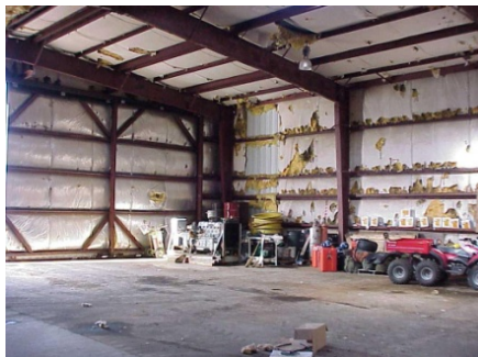
Interior of Hangar
