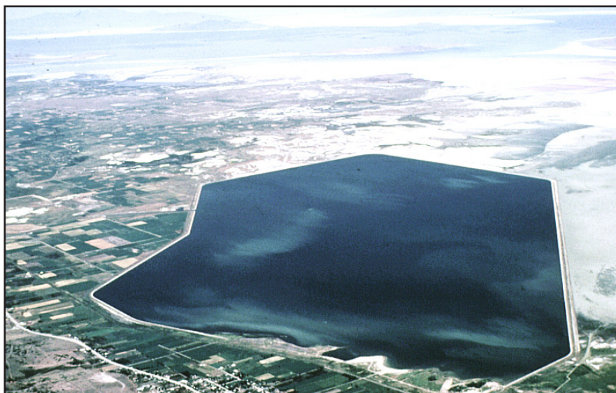
An aerial view of Watkins Dam.
