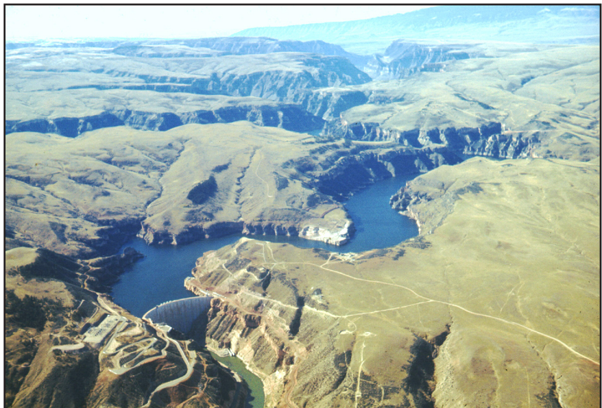
Aerial view of Yellowtail Dam on the Bighorn River.
