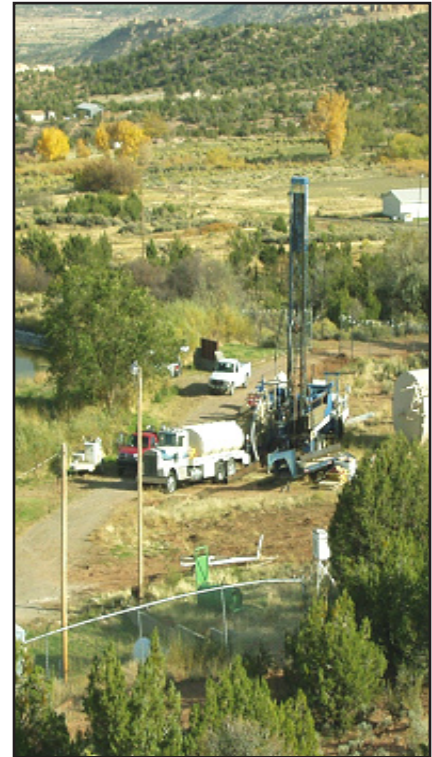
This 452-foot-deep well produces 8 to 20 gallons per minute of nonpotable water for Toadlena Fish Hatchery.
