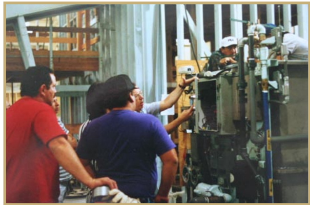
Hands-on-training of Tribal Water Treatment Plant operators by Reclamation Water Treatment Engineering and Research staff on the Green Sand Filter Unit, designed by Reclamation.
