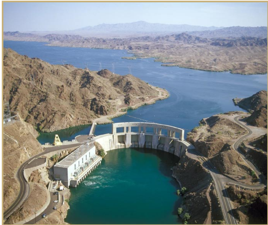
Parker Dam, located on the Colorado River northeast of Parker, Arizona.
