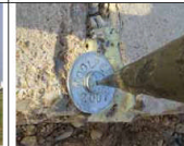
Photograph Type #4 (Close-in). Close-up photo depicting nail, washer and markings.
