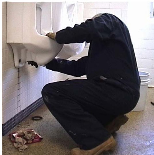
Figure 1: Pipe-fitter in awkward posture
