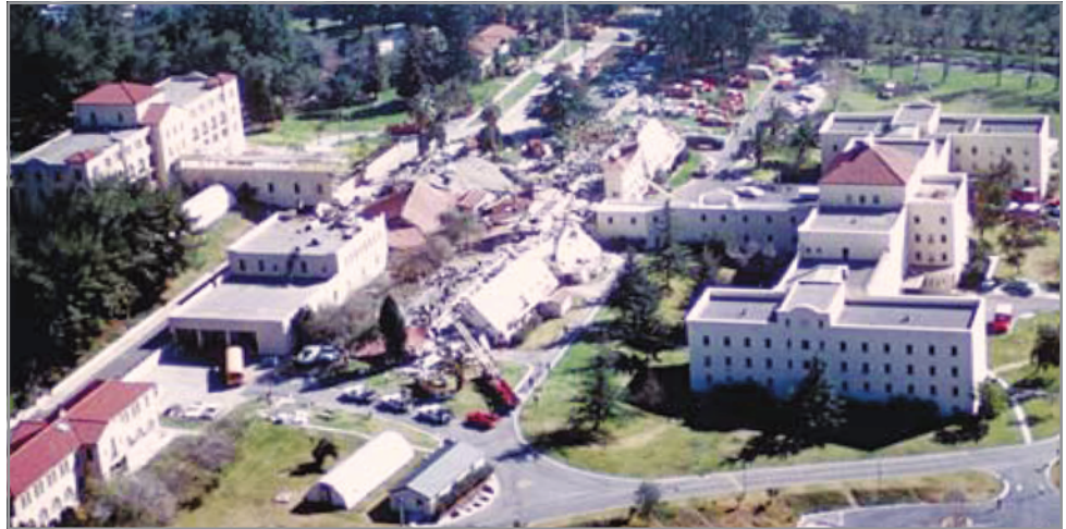
The 1971 San Fernando, California, earthquake (magnitude 6.7) collapsed four buildings at the San Fernando VA Hospital, killing 49 people. The buildings had been built in 1925, before building codes were in effect. Real-time seismic monitoring of such buildings can provide critical information about their structural integrity and help save lives in future earthquakes.
