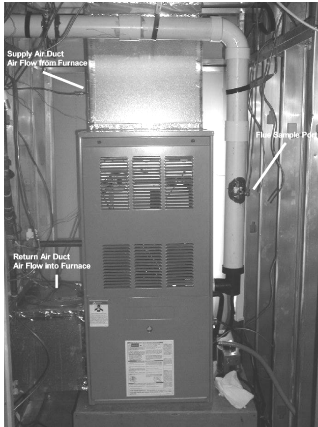
Figure 2.1. High Efficiency, Induced Draft Test Furnace
