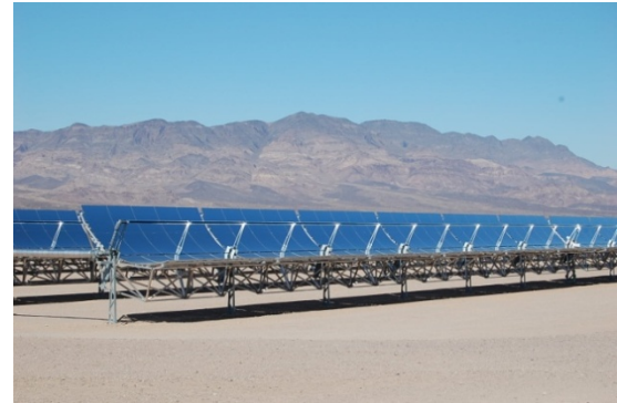
Figure 5-1. Example of a Parabolic Trough Plant
