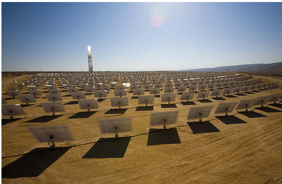
Figure 5-5. Example of a Power Tower and Heliostat Array
