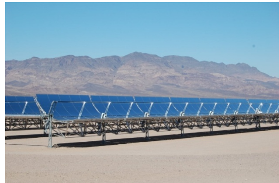
Figure 5-1. Example of a Parabolic Trough Plant
