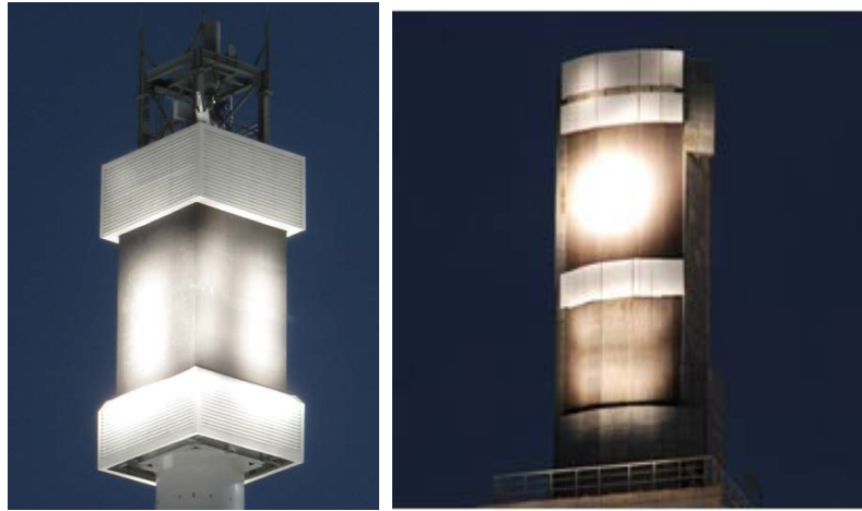
Figure 5-6. Examples of Direct Steam Receivers in Operation
