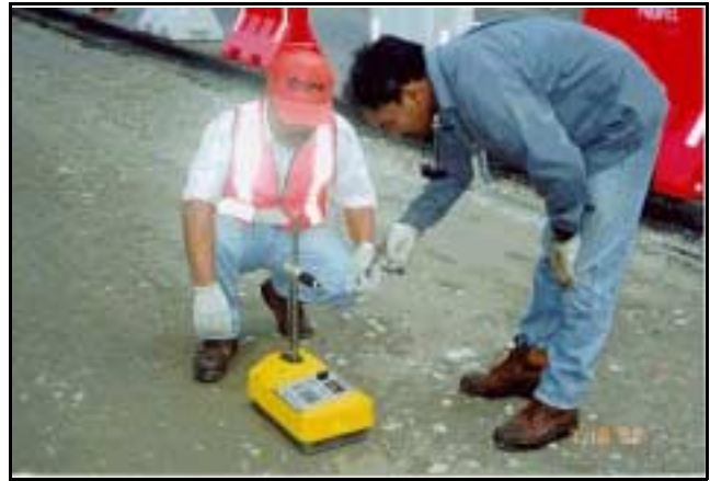
A typical moisture-density gauge in use.
