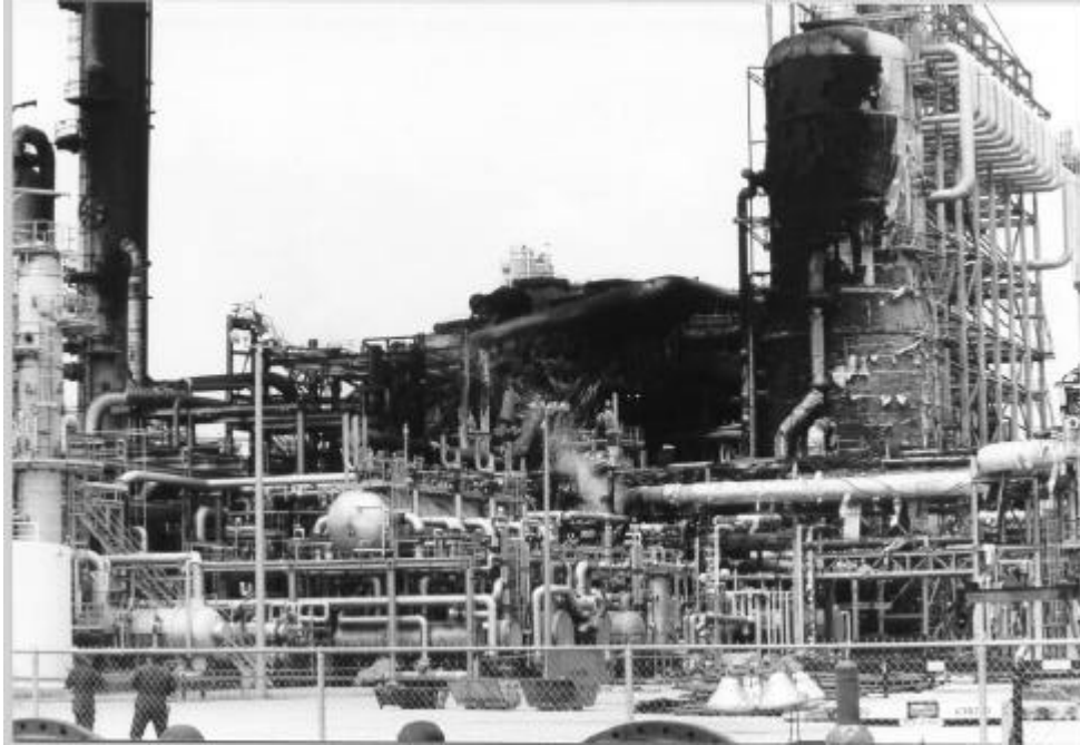
Figure E-1: Photograph of the damage resulting from the explosion and fire at Shell Olefins Plant Number 3 (view from west of blast area). Note the heavy structural damage in the rear center of the photograph.
