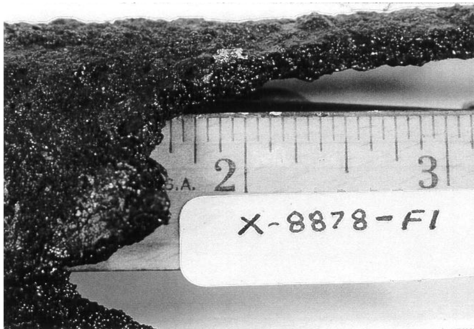
Figure E-22: At higher magnification, this macrograph shows the high temperature oxidation and fire damage around the opening in the pipe section. Laboratory analysis of this and each of the other three pipe sections revealed similar fire-induced failure modes, indicating that none were the likely source of the initial flammable gas leak.
